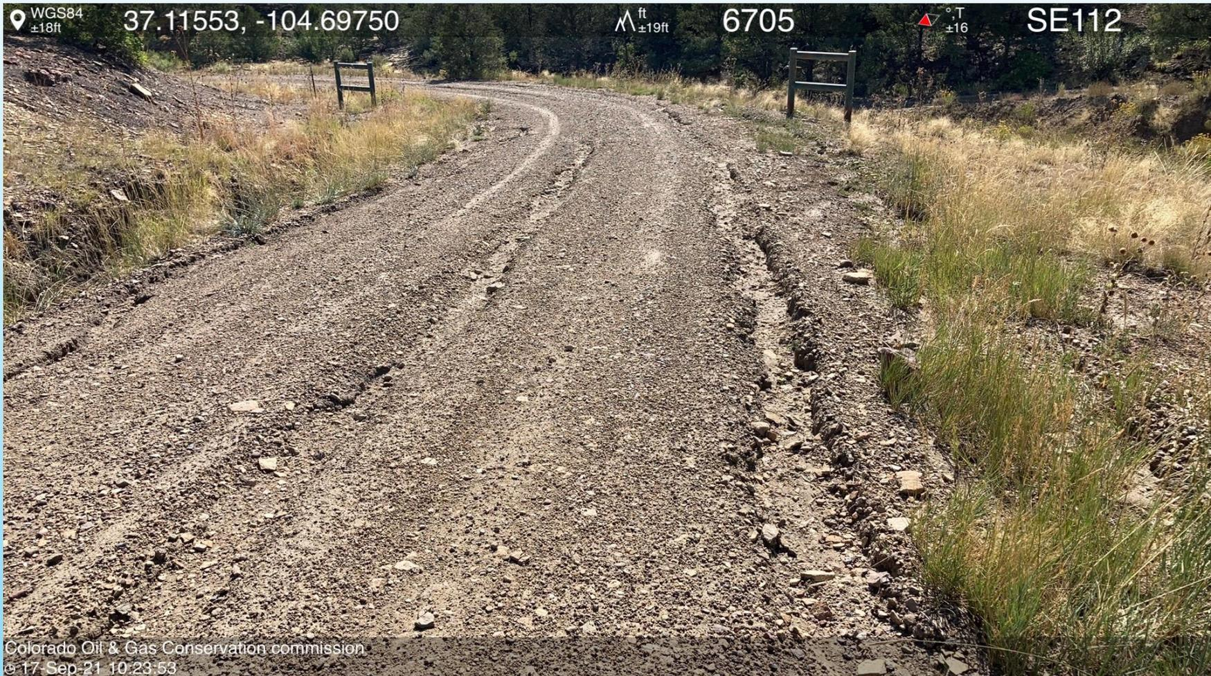
**PHOTO 4: VEHICLE RUTTING AND STORMWATER EROSION OCCURING ON ROW NEAR LOCATION.
