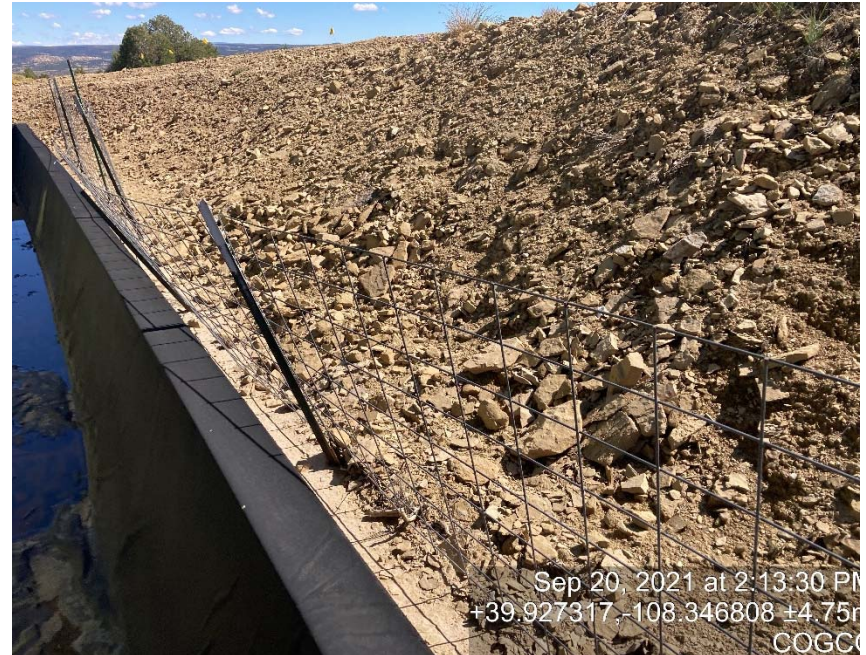
Lack of stabilization/erosion
