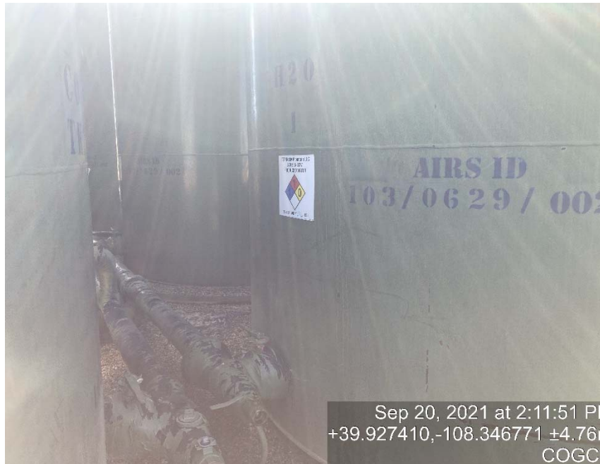
Tank labels missing quantity
