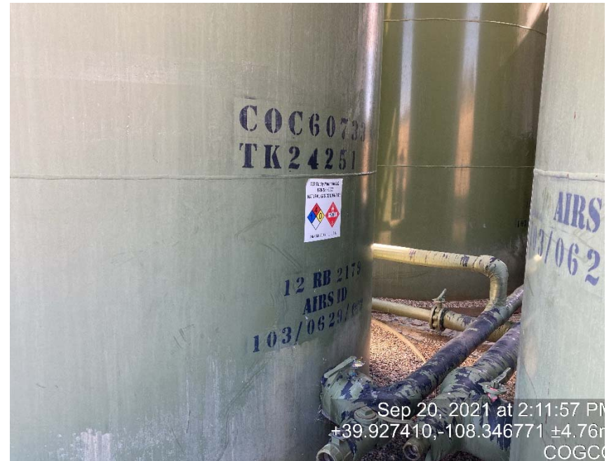
Tank labels missing quantity
