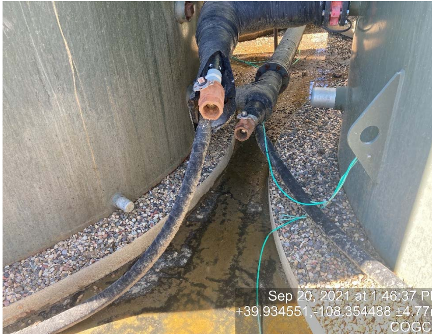
Missing plugs/caps load out lines
