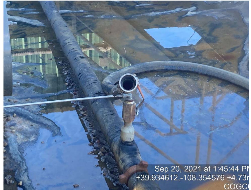
Missing plugs/caps load out lines
