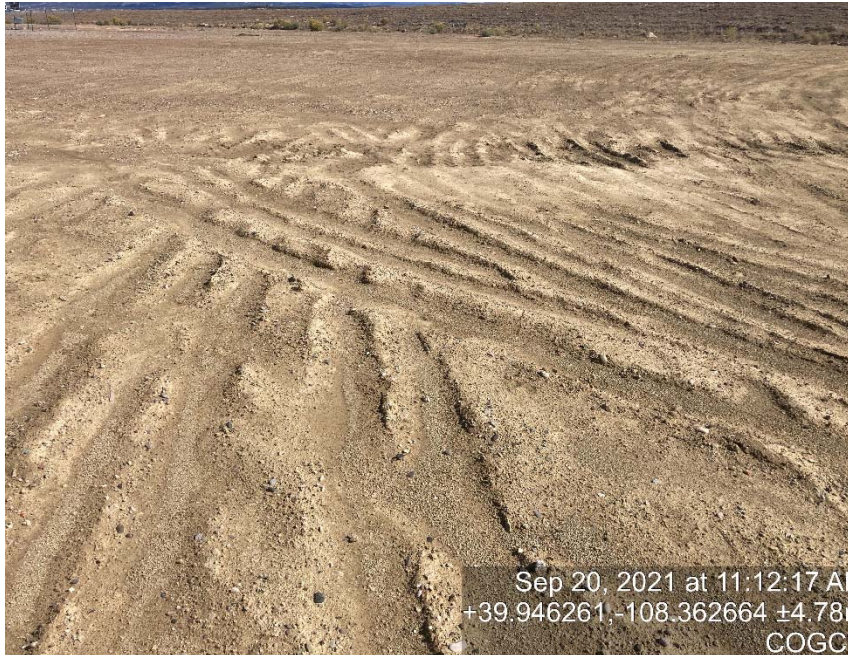
Lack of stabilization/compaction
