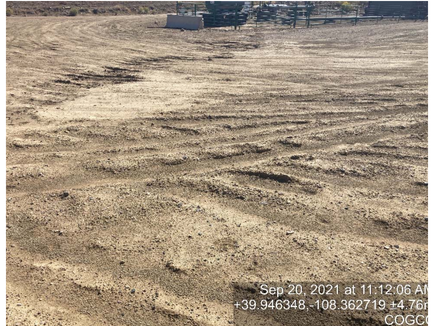
Lack of stabilization/compaction
