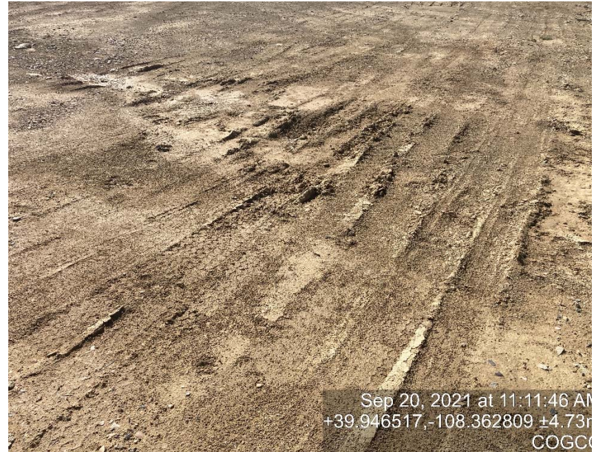
Lack of stabilization/compaction
