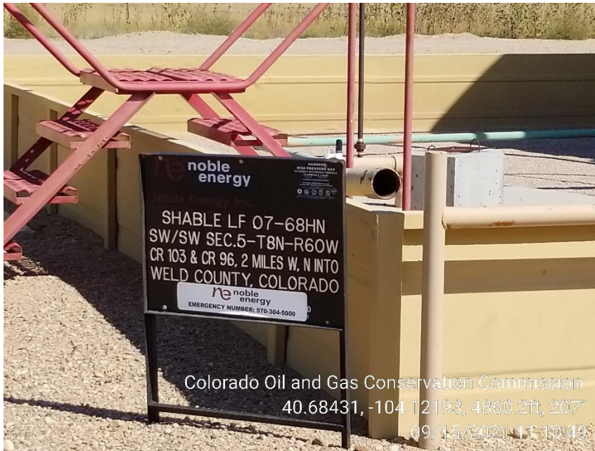
Photo 5 – Tank Battery Sign
