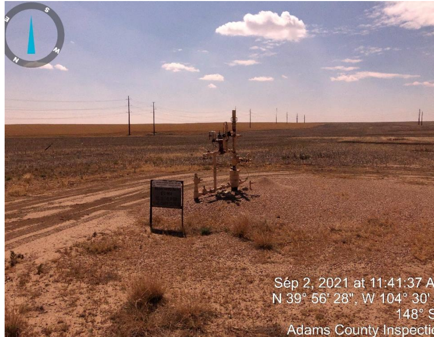
Photo #3 Well Head.
