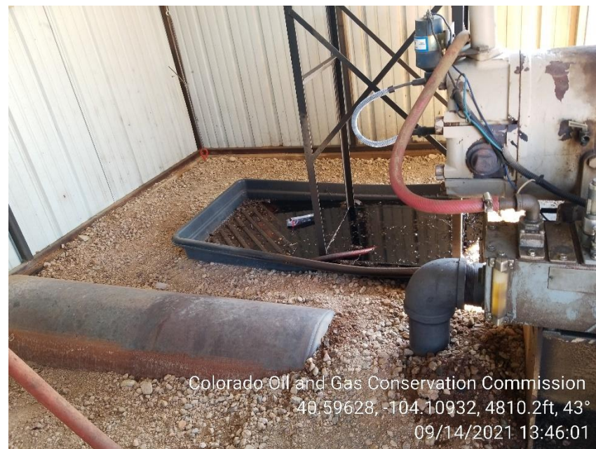
Photo 4 – Oily Waste at Gas Engine
