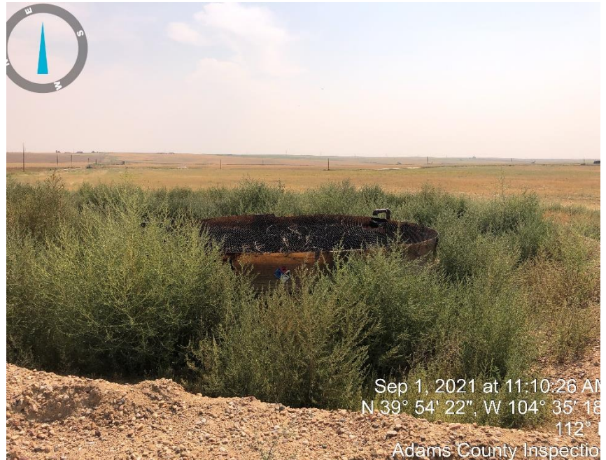
Photo #2 open top tank.
