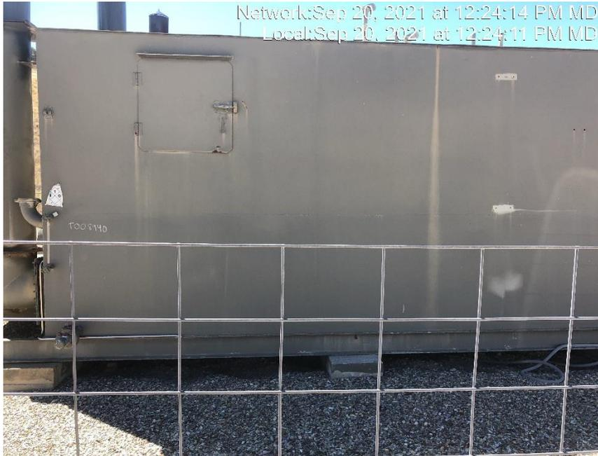
**Photo #4916 Glycol storage tank missing required information.**
