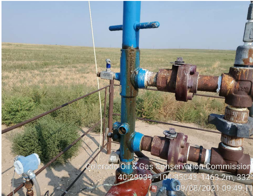
Lubricator leak on 9/8/2021
