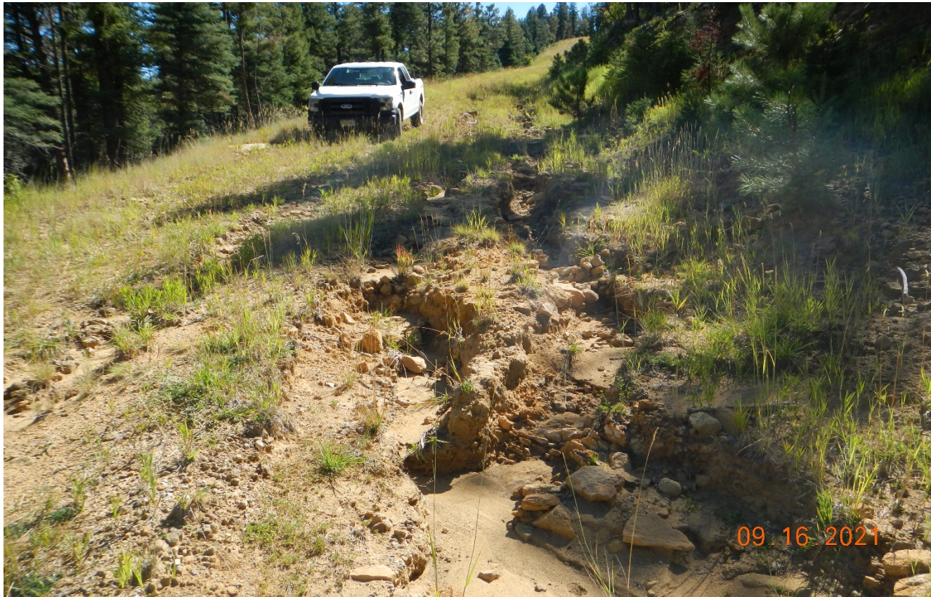
Photo 8. Facing northwest along the access road descending into the canyon. There is erosion along the road all the way down to the canyon bottom.
