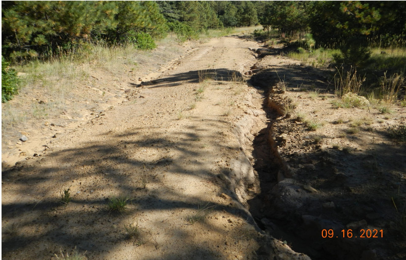
Photo 3. Facing northeast further along the access road. The road is not stabilized and there is erosion channels along the road.
