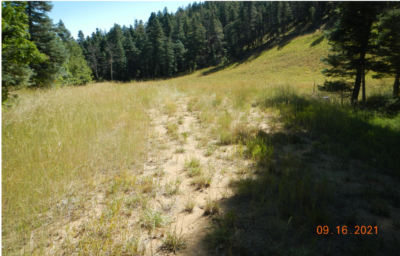
Photo 11. Facing southeast toward the location. There is a culvert that remains at red arrow. The location has been recontoured and reclaimed.
