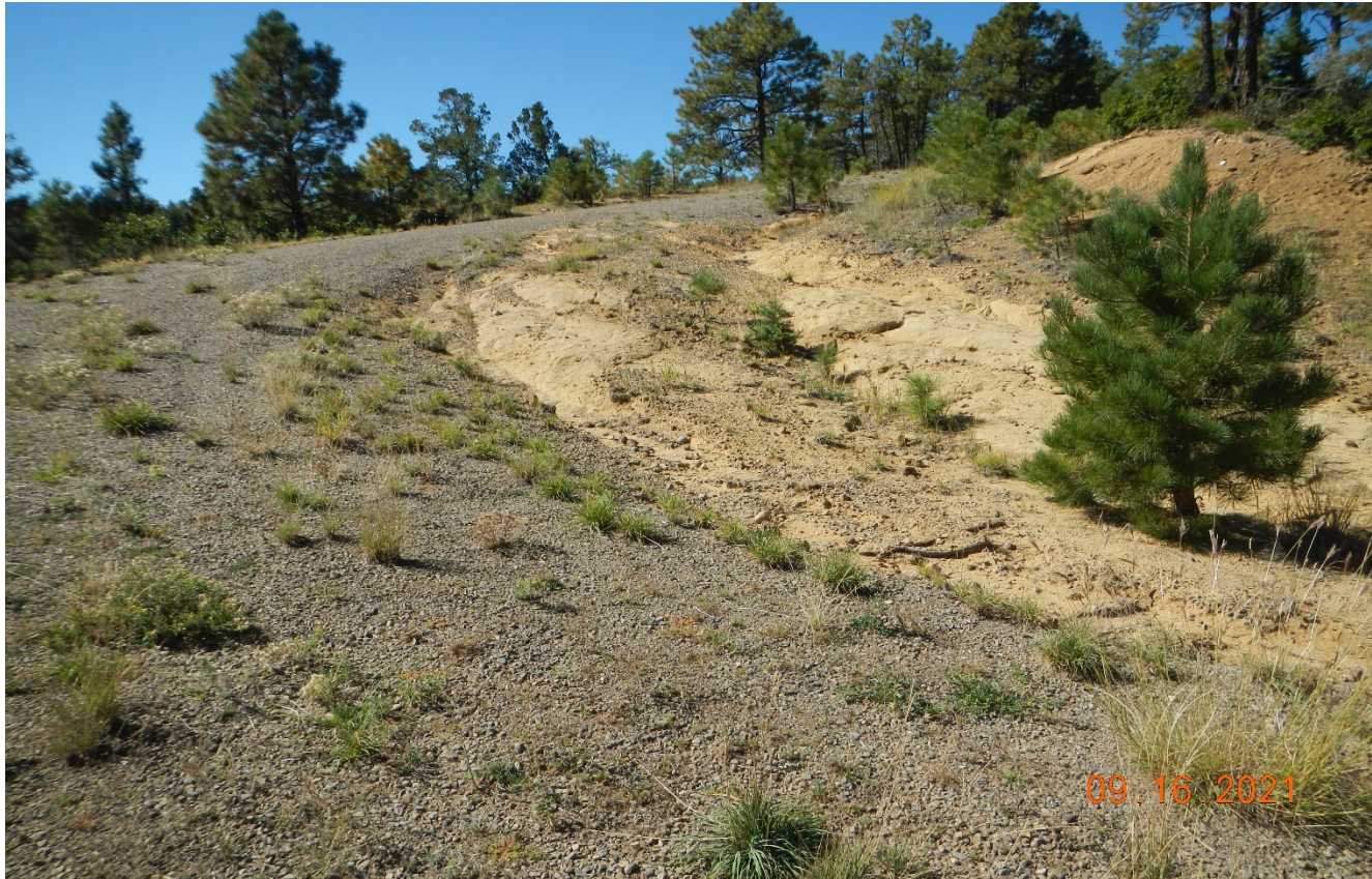
Photo 4. Facing back where the road turns down the hill side into the canyon. The side of the road is not stabilized in this area.
