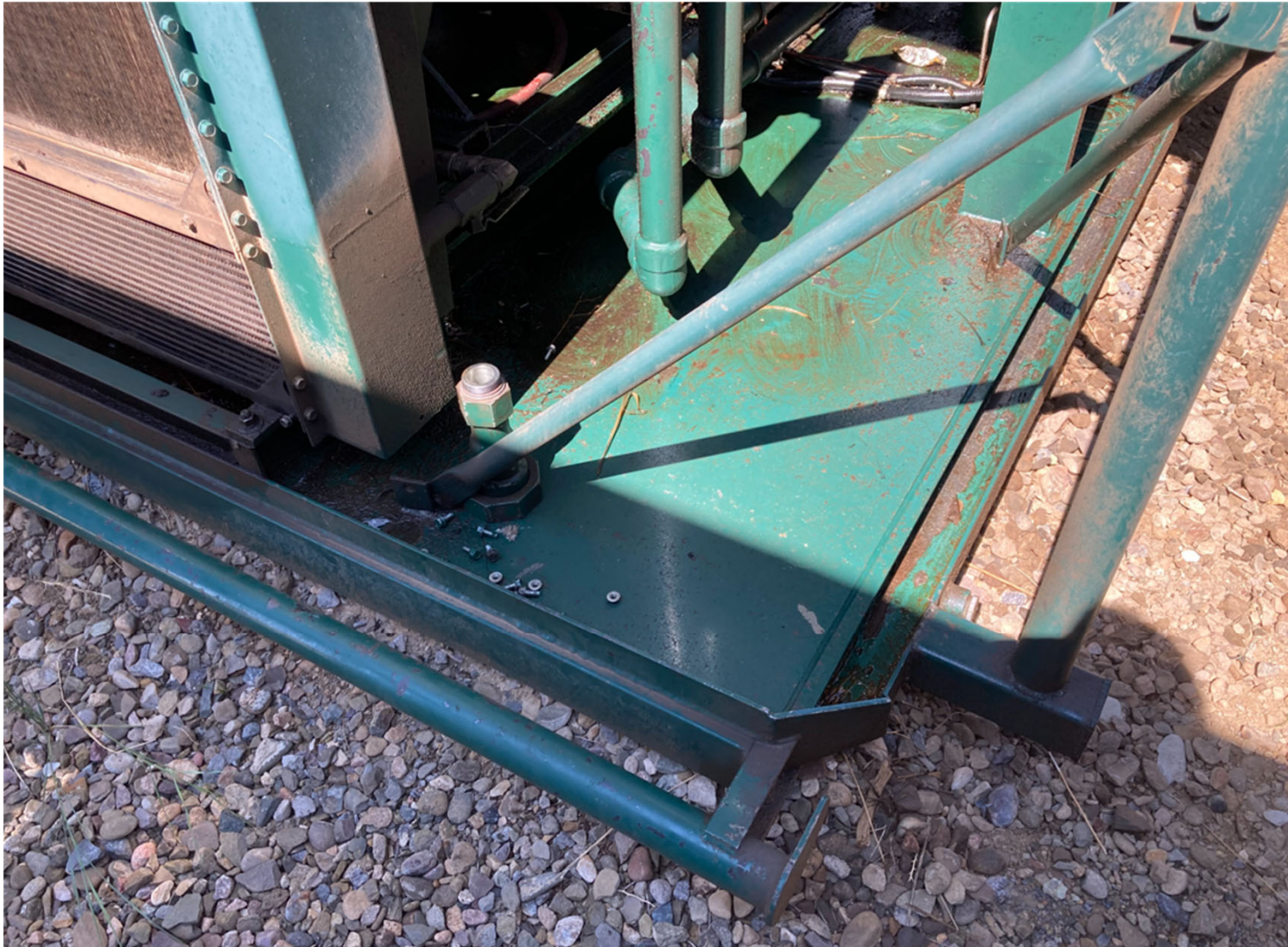
PHOTO 2: THE OIL ABSORBENT PADS WERE REMOVED FROM THE SKID.
