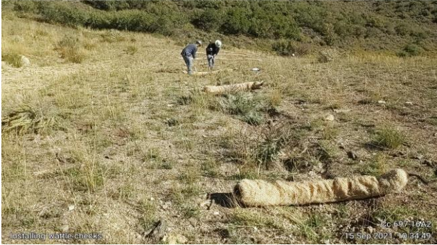
Installing Additional Excelsior Wattle Checks
