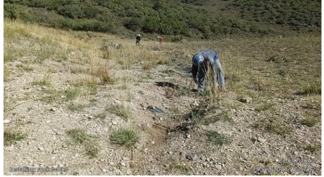
Maintaining Existing Rock Sock Checks
