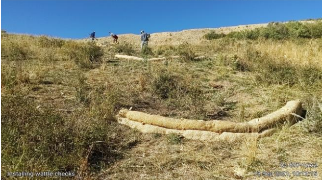
Installing Additional Excelsior Wattle Checks to Provide Additional Protection during Runoff
