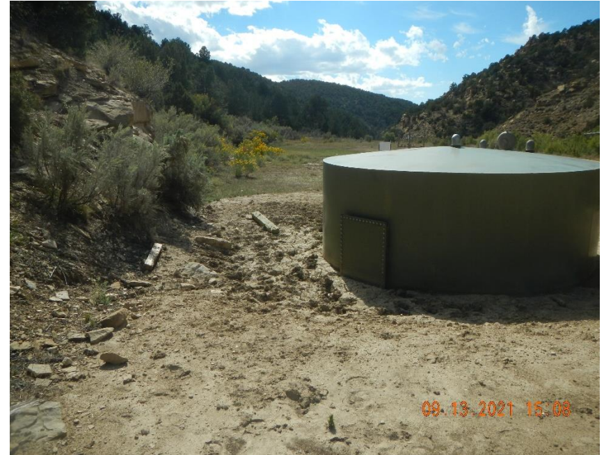
Tank berm and base not maintained.
