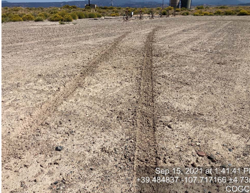
Lack of stabilization/compaction
