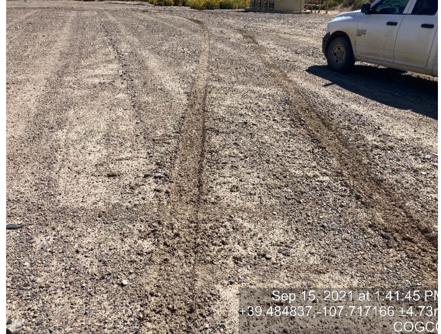
Lack of stabilization/compaction
