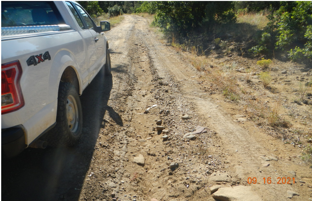
Photo 3. Stormwater erosion is occurring further along the road as well.
