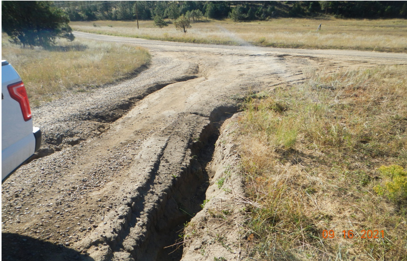
Photo 2. Stormwater erosion of the access road is directed down toward the County Rd.
