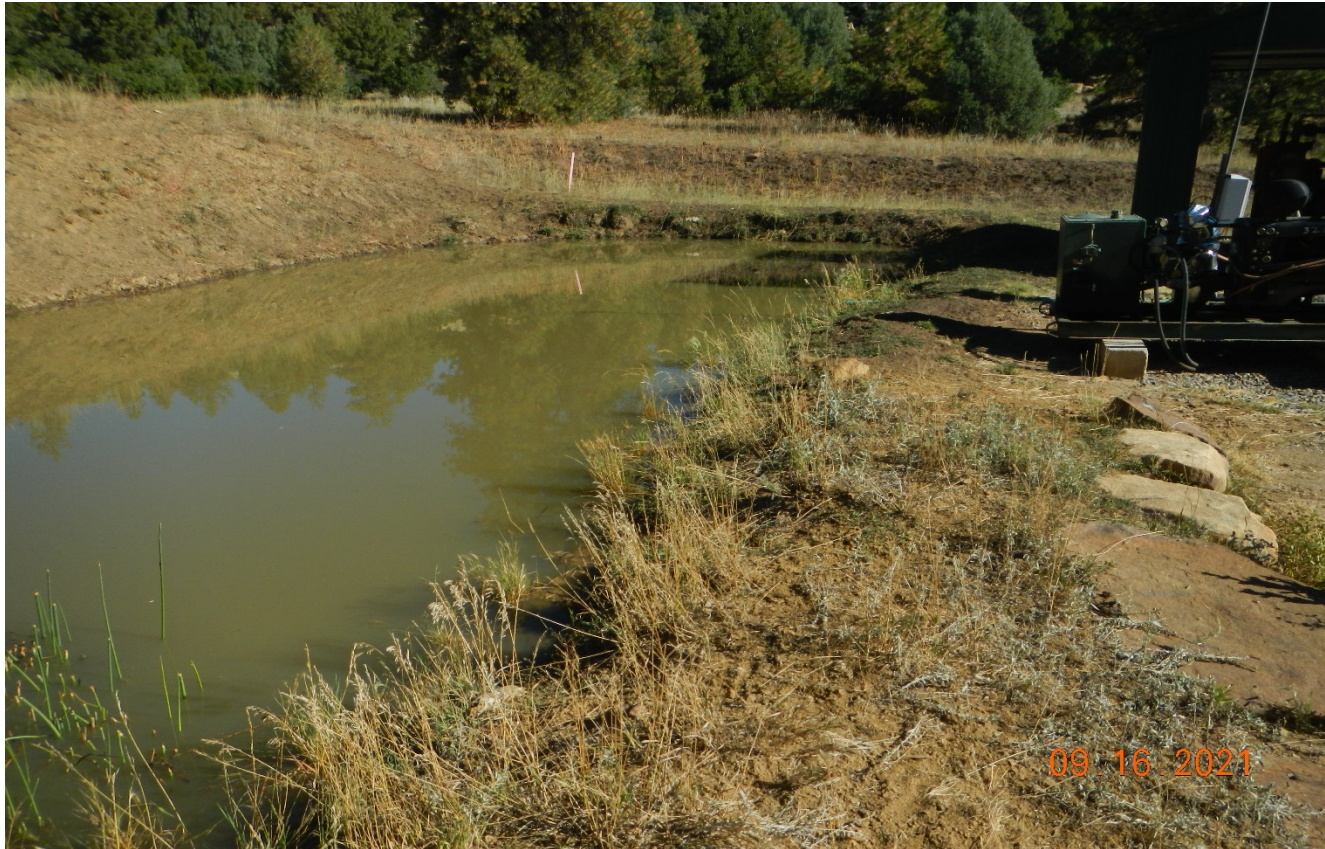
Photo 5. The water level is above freeboard at the pit.
