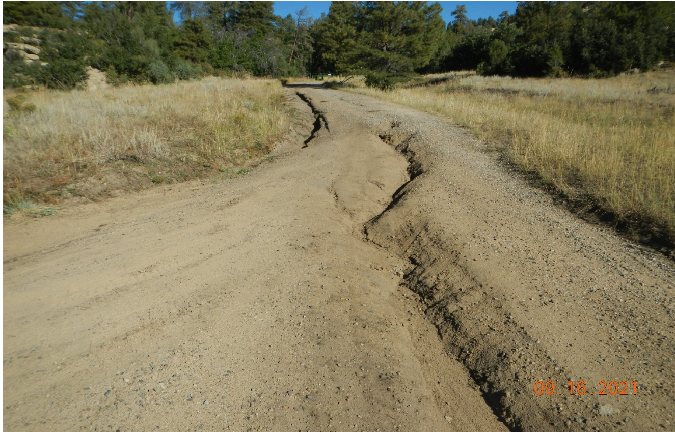
Photo 1. Facing northwest toward the access road. There is erosion along the road that needs to be repaired and stabilized.
