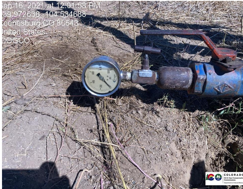
Pic 1 casing valve
