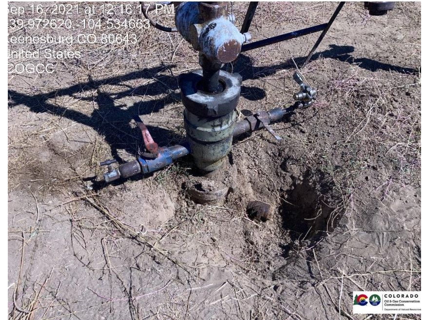
Pic 2 Bradenhead exposed unable to open bradenhead valve.
