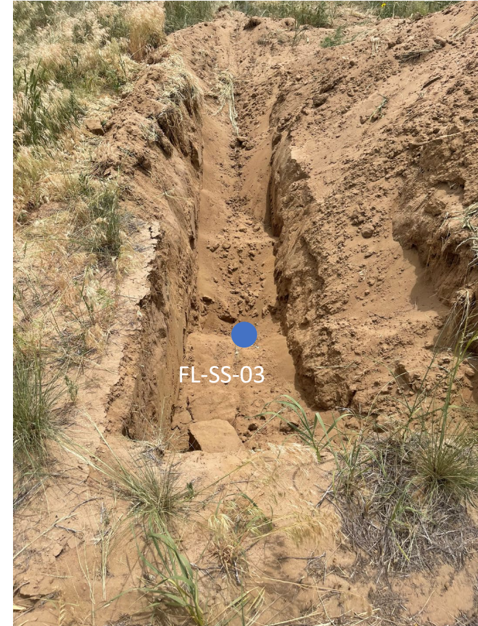
Flowline removal Bellholed/pulled prior to assessment No petroleum hydrocarbon staining or odor observed Screening sample collected: FL-SS-03 @ 3.5' = 1.6 ppm-v
