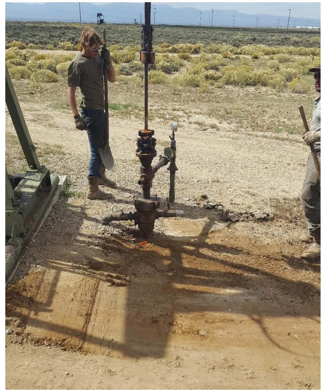
Figure #1 bradenhead access has been installed.
