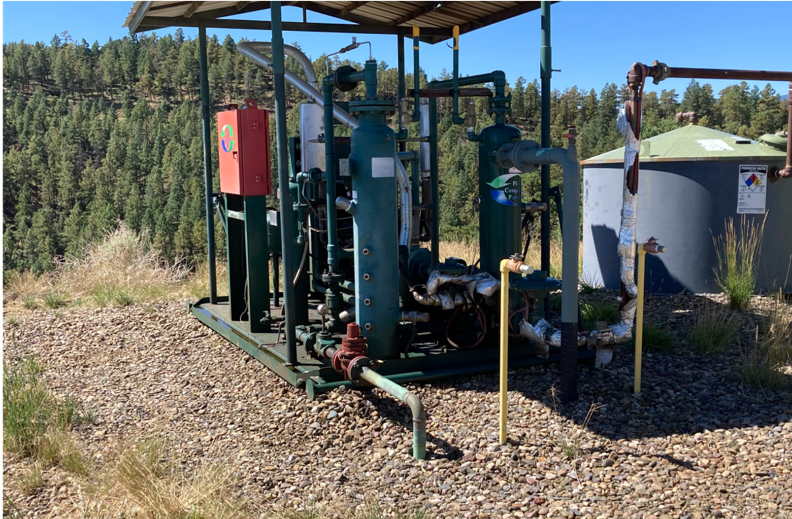
PHOTO 1: MAINTENANCE WAS CONDUCTED TO THE LIQUID RING COMPRESSOR TO STOP THE OIL LEAK. THE IMPACTED SOIL/GRAVEL NEXT TO THE LIQUID RING COMPRESSOR WAS REMOVED FROM THE LOCATION. SELF INSPECTION PROCESS WAS REVIEWED.
