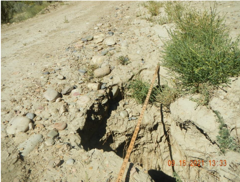
Sink hole in shoulder of access road. Just south of DTU 1056 entrance.
