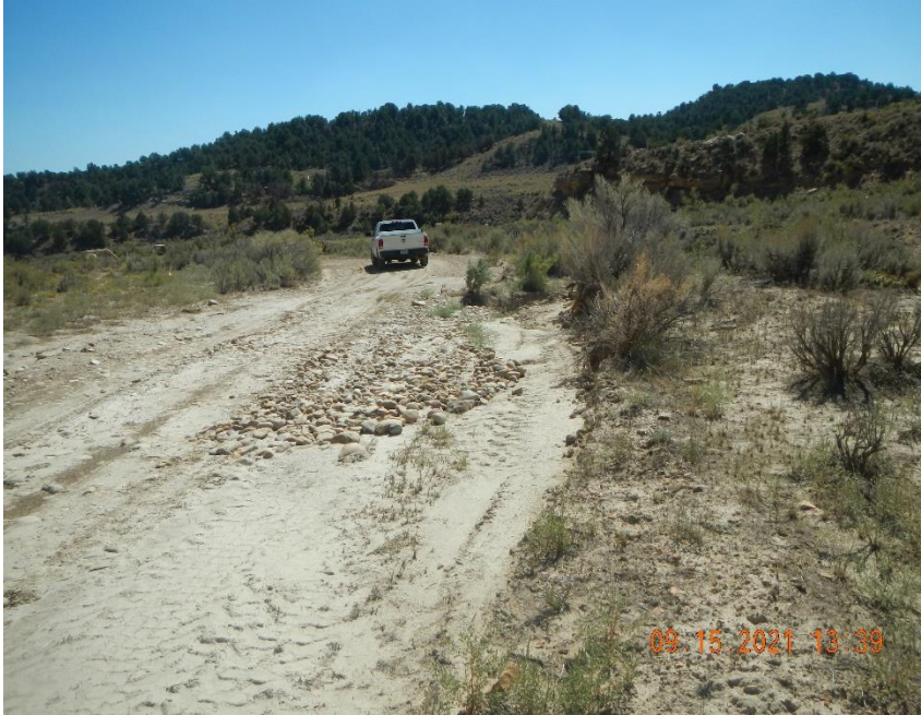
Storm water erosion of access road.
