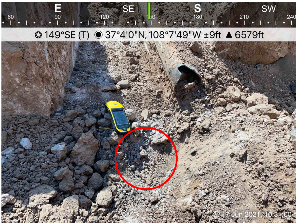
Photo 4: SS04 collected a flowline segment at the Ferguson No. 2 (OWP) F-12, 6/17/2021.
