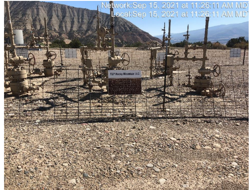
Photo #4880 Wellhead sign weathered and not legible.
