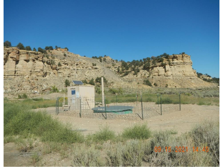
Dead weed debris covering location.
