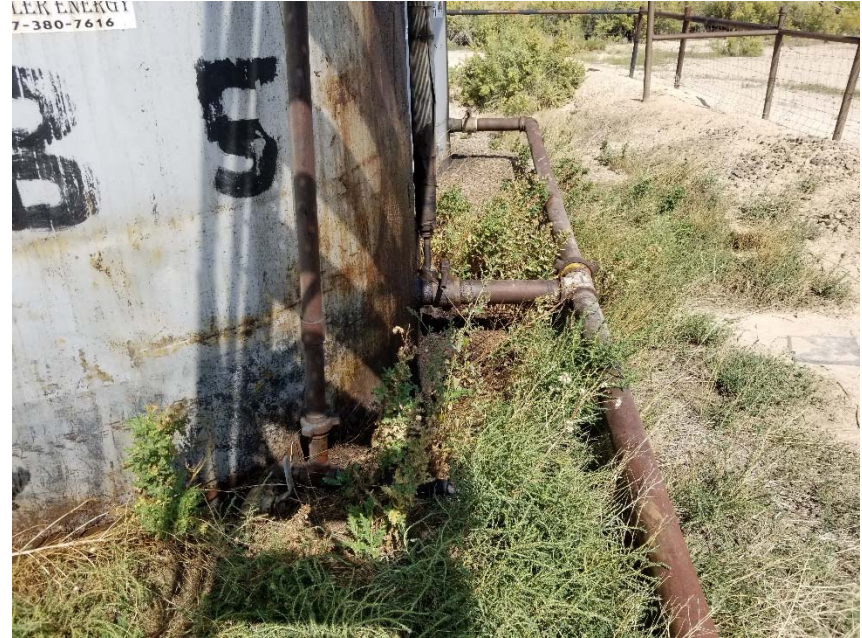
Photo 4. Stained soil at tank bases.
