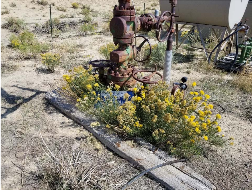
Photo 3. Wellhead sign obscured by vegetation. No bradenhead access apparent.
