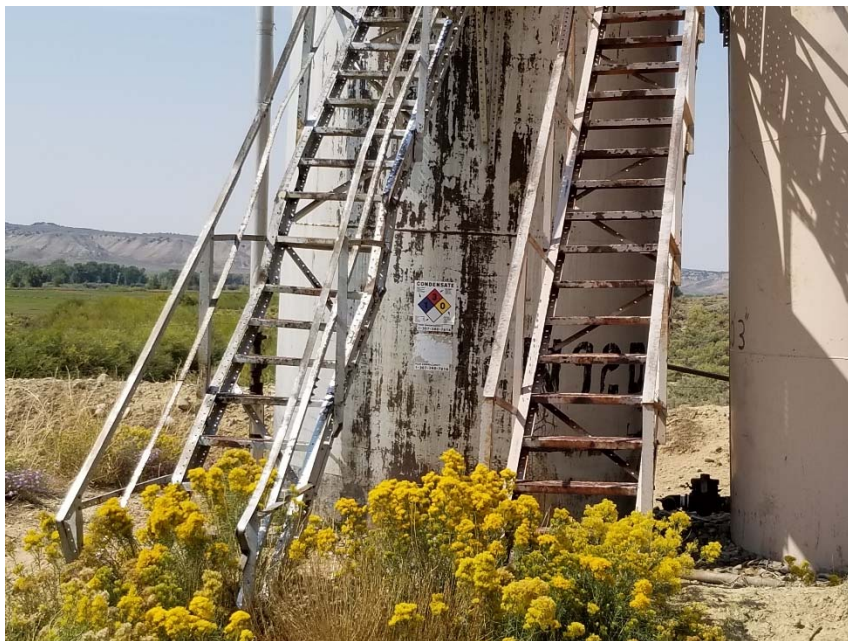
Photo 7. Incomplete tank label.
