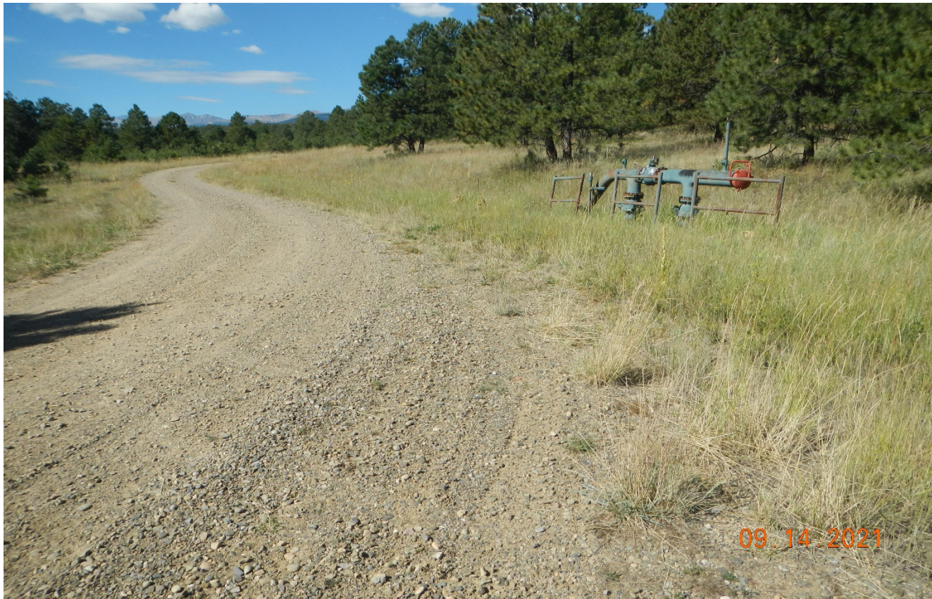
Photo 1. Facing west along the access road. The pig launcher receiver has not been removed.
