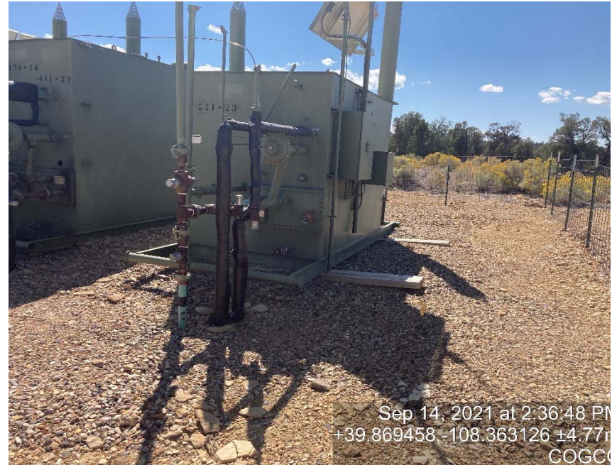
Lack of labels on glycol storage vessels
