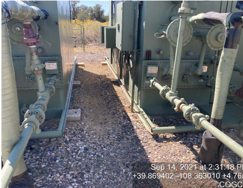
Lack of labels on glycol storage vessels
