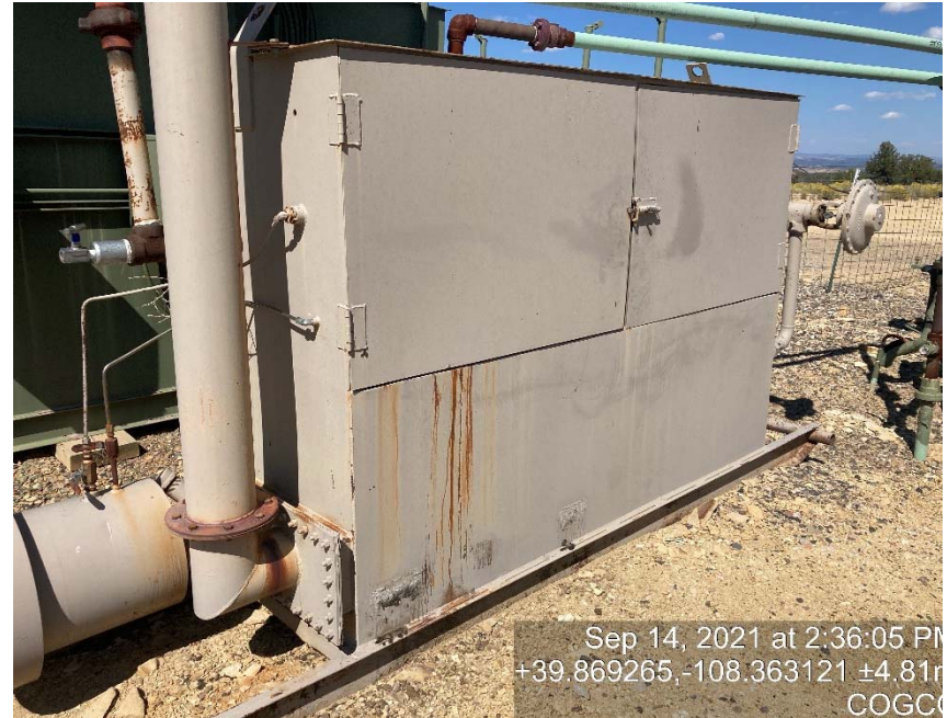
Lack of labels on glycol storage vessels
