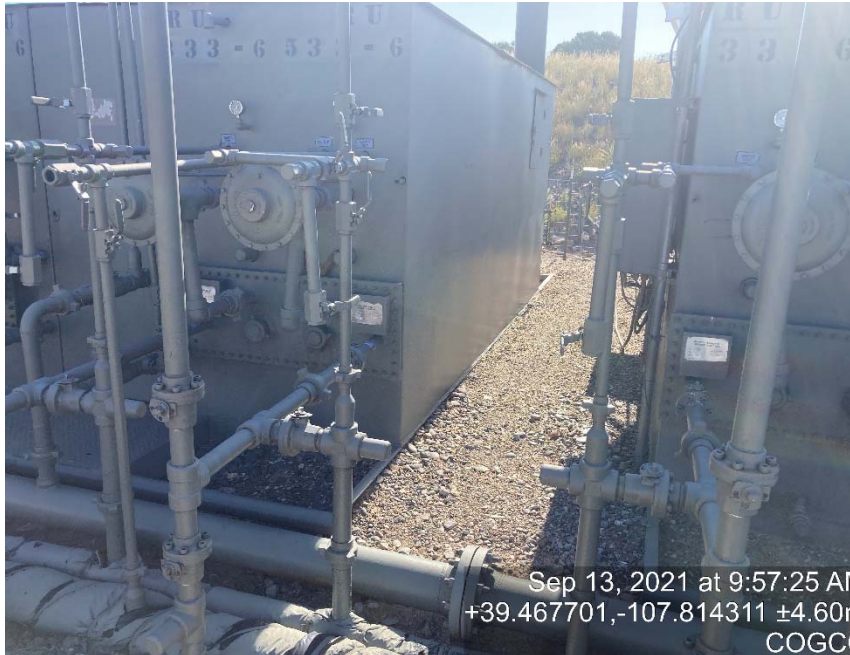
Glycol vessel missing labeling
