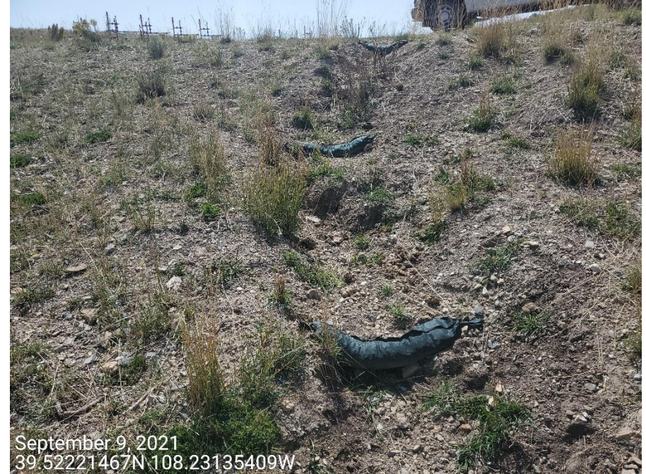
Photo 3: Photos taken from the northern interim area. Photos show gully erosion degradation due to runoff from the Location. Rock-socks observed within the channel. Stormwater and erosion control measures observed are inadequate alone to control runoff from the Location in a manner that minimizes erosion and site degradation.
