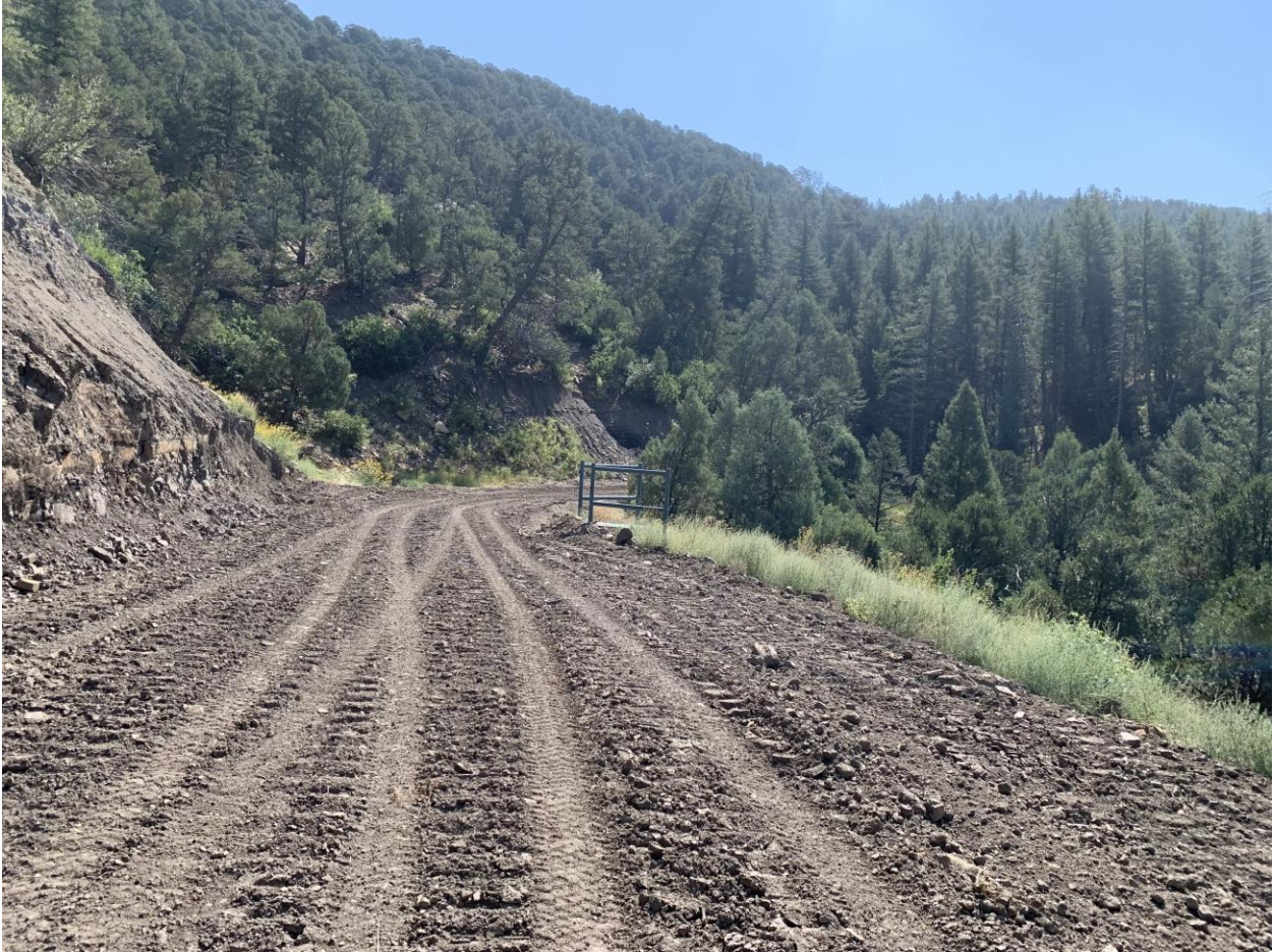
Installed and repaired required BMPs per Rule 1002.f.(2) C.
