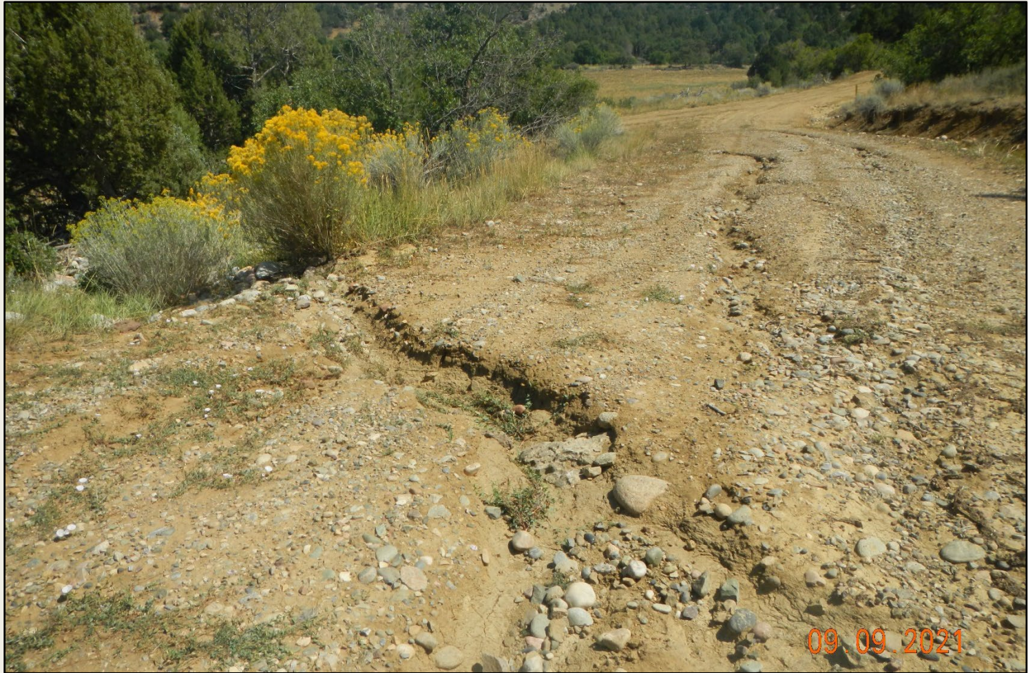
Photo 4. View of erosional channel shown in Photo 2, where it flows downslope eroding the access road surface and flowing off of the project area.
