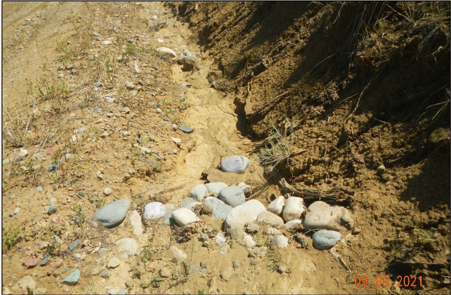
Photo 5. View of cobble BMPs along the southern project area that are full of sediment and not functioning, or adequate for this area. .
