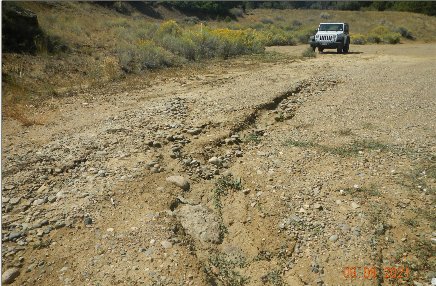
Photo 3. View of erosional channel forming on the well pad and flowing down the access road (facing upslope).
