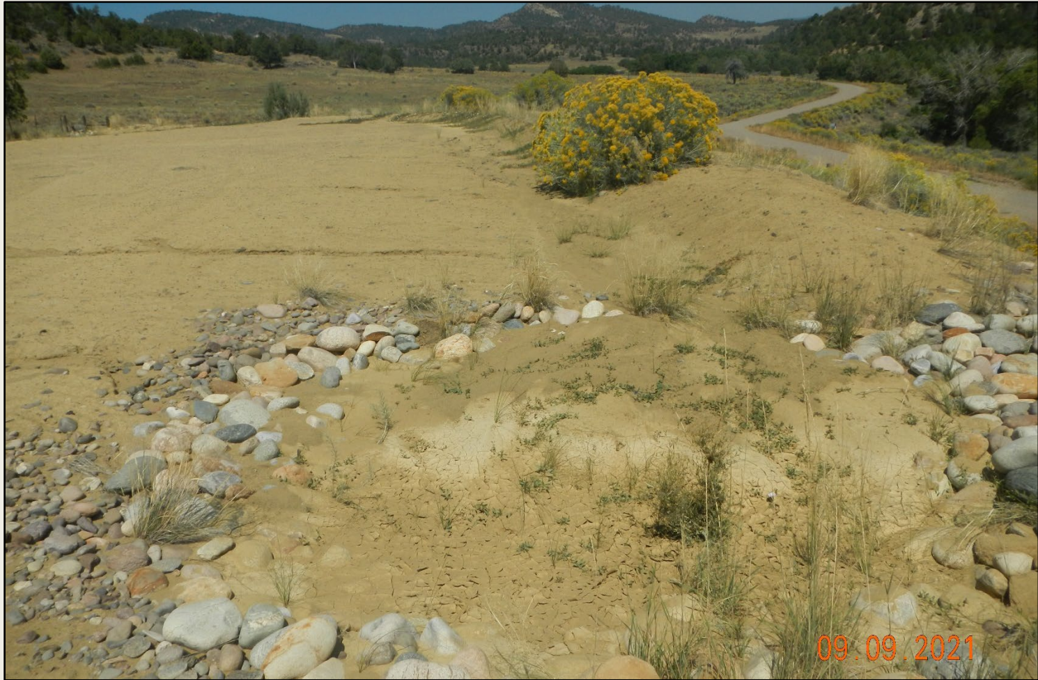
Photo 3. View of sediment deposition within the eastern sediment trap, largely full and needing maintenance.
