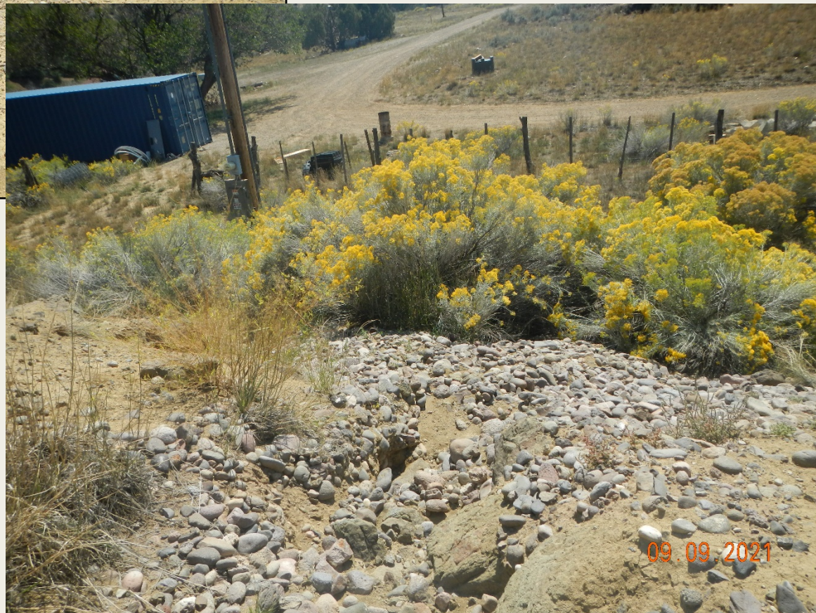
Photo 2. View of erosional channel on the well pad (left) and cobble BMP eroded and displaced on the fill slope (right).
