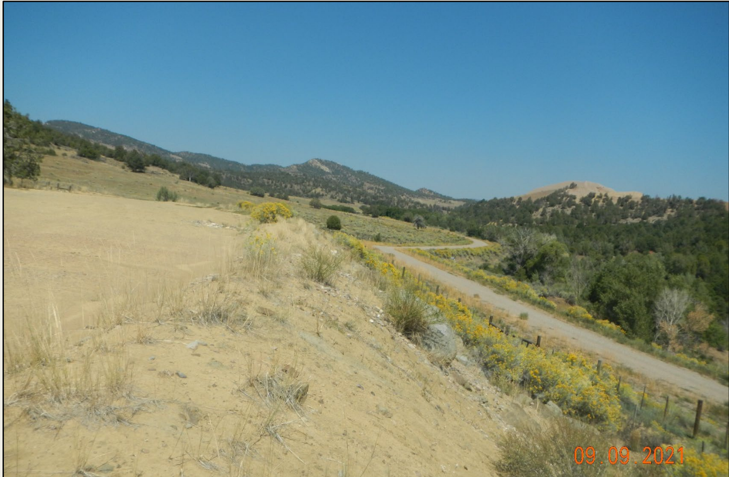
Photo 4. View of the eastern fill slope from the southeastern corner facing northward. Revegetation is progressing in portions of the fill slopes with rubber rabbitbrush, sand dropseed, and crested wheatgrass. Other portions remain bare and eroding and need spot seeding and stabilization.
