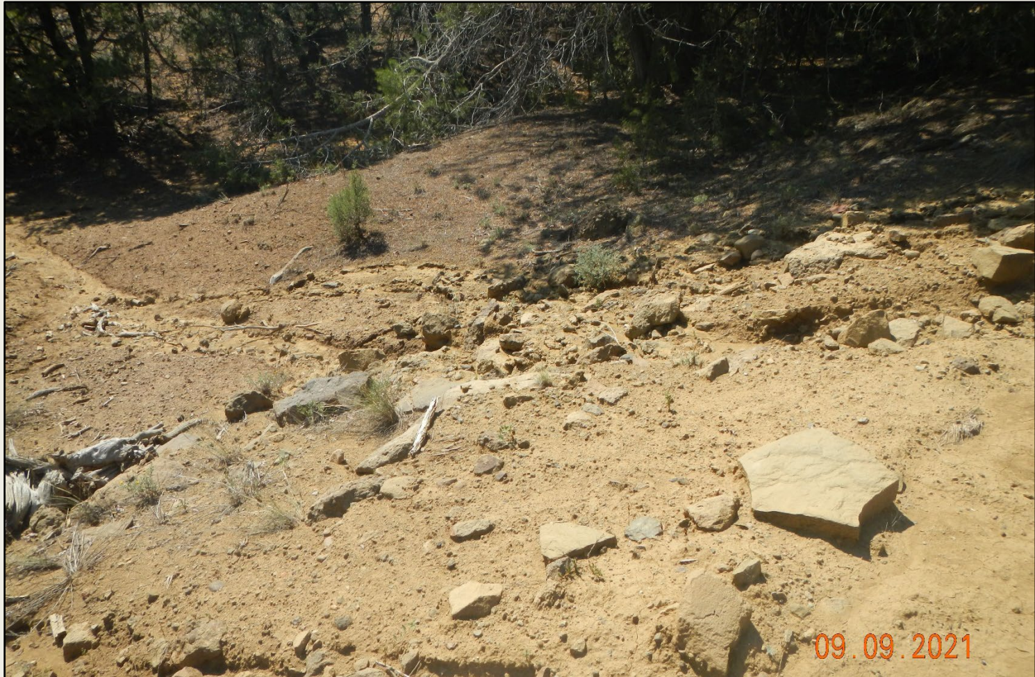
Photo 7. View of area (facing downslope) on the access road where stormwater flows are flowing down fill slope and eroding/carrying sediment offsite. Fill slope is not stabilized.
