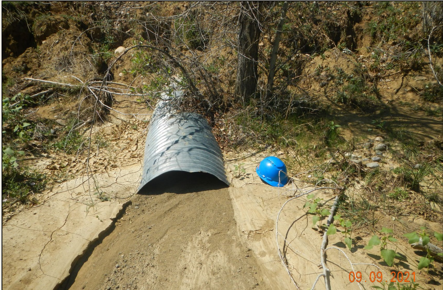
Photo 11. View of culvert outlet at stream crossing. Approx 3-ft culvert is full of sediment and not adequate to convey stormwater flows.
