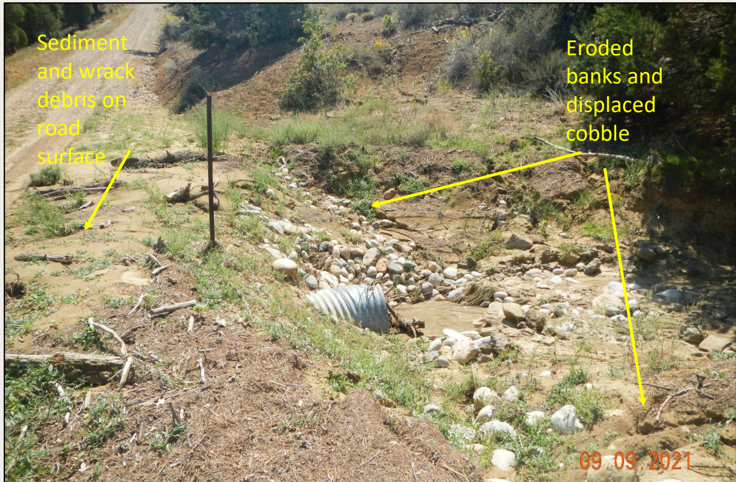
Photo 9. View of upstream side of culvert crossing where cobble is displaced, banks eroded, and sediment/wood wrack is settled on road surface.
