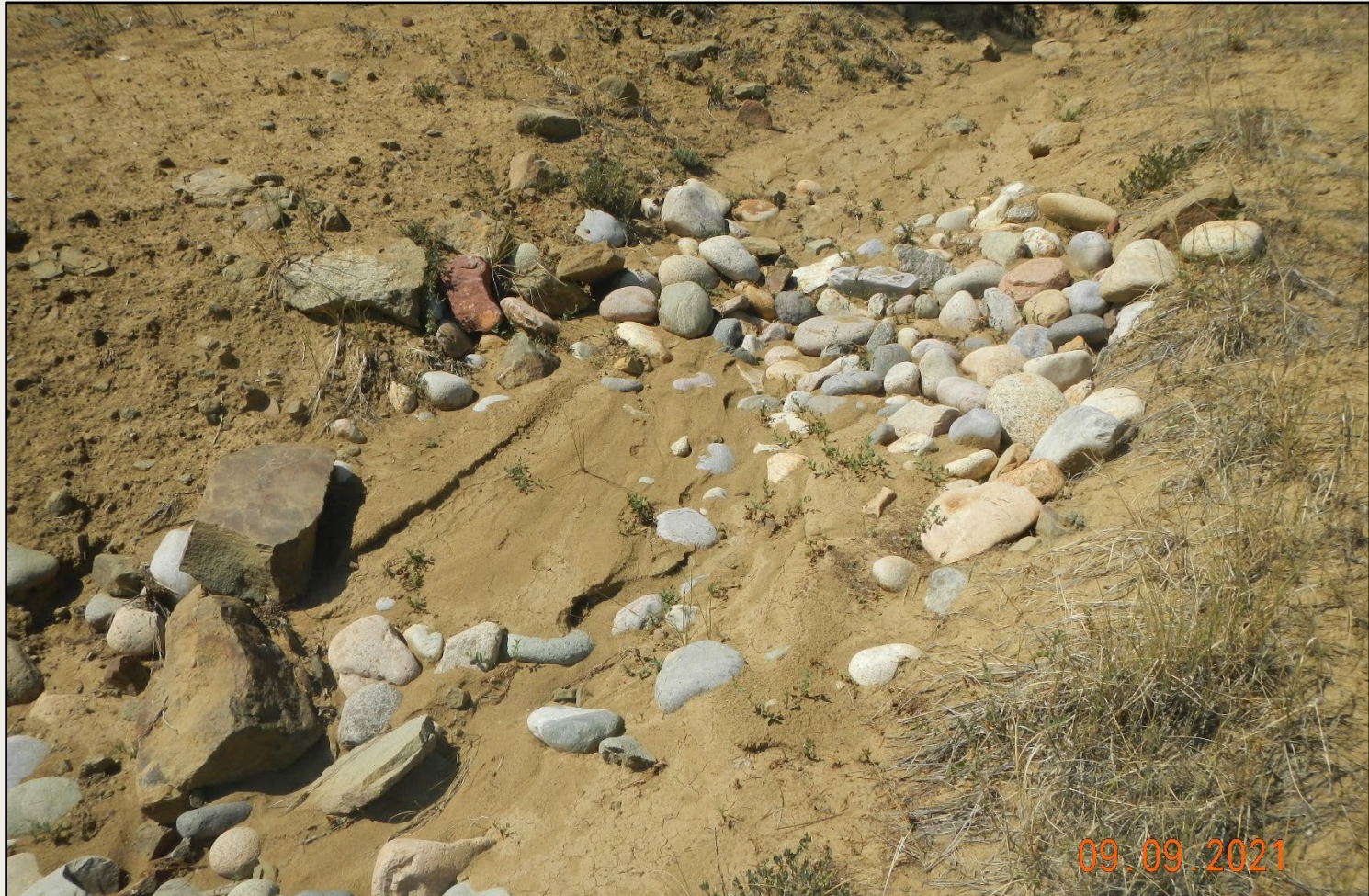
Photo 5. View of stormwater BMPs in the southeastern project area, that are full of sediment and eroding. BMPs do not appear adequate.
