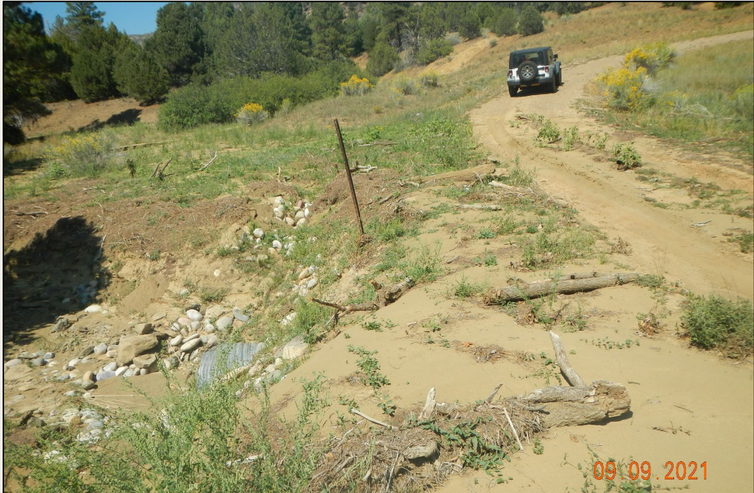
Photo 10. Another view of upstream side of stream crossing with wood wrack and sediment discharge observable in the foreground.
