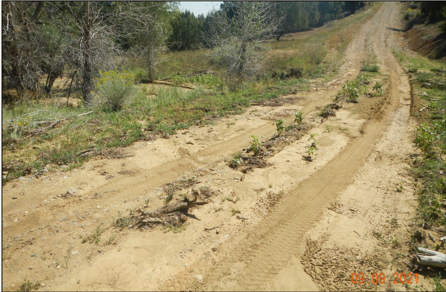
Photo 8. View of stream crossing along access road where stormwater flows are flowing over the crossing resulting in erosion and sediment discharge. Crossing is not properly designed to contain stormwater passage.
