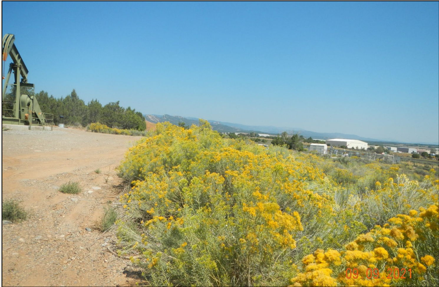
Photo 2. View of the eastern fill slope from the southeastern corner facing northward. Revegetation is progressing with western wheatgrass, rubber rabbitbrush, and smooth brome.
