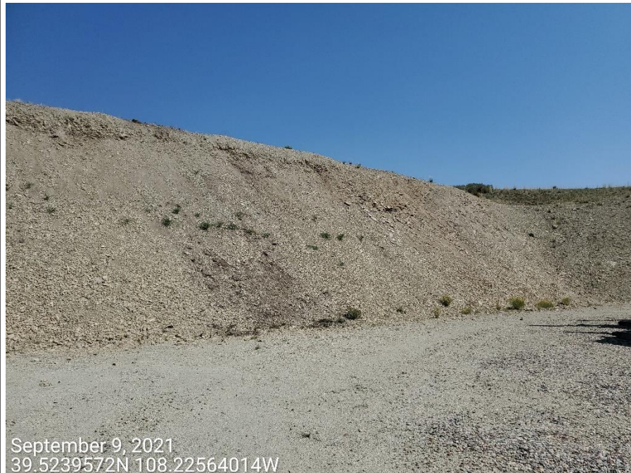
Photo 3: Photos shows example of the cut slopes, where BMPs to protect and stabilize the slopes are missing or insufficient on the Location.
