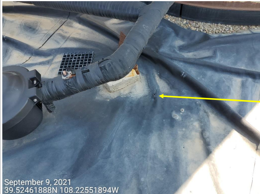
Photo 5: Photos show tear observed in the liner on the north side of the tank battery
