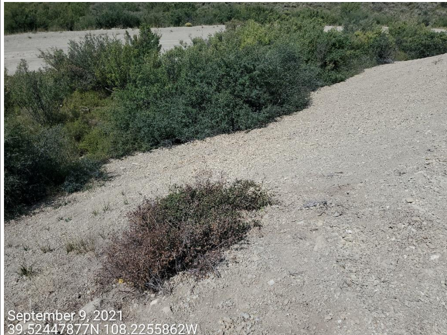
Photo 6: Photos shows control measures are missing or insufficient to protect and stabilize the fill slopes, and manage runoff on the northwest end of the Location.
