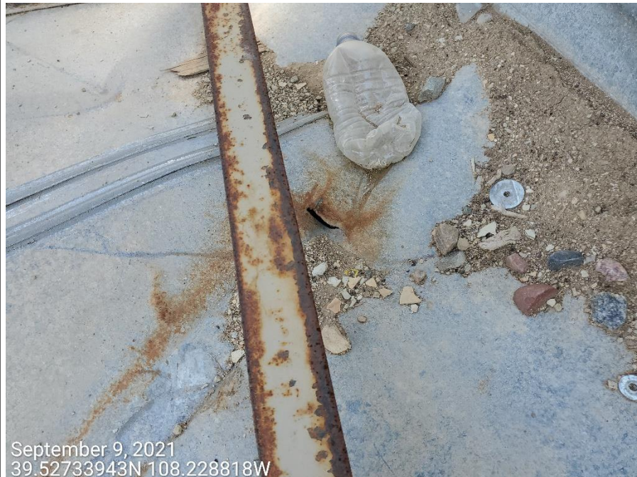
Photo 8: Photo taken from the containment BMP for the tank in left-photo 6. Photo shows multiple punctures observed at the base of the BMP.
