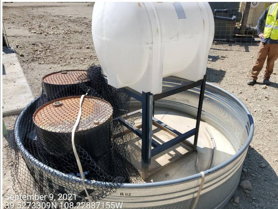
Photo 7: Photos provide examples showing that wildlife protection devices are missing or insufficient at several secondary containment BMPs.
