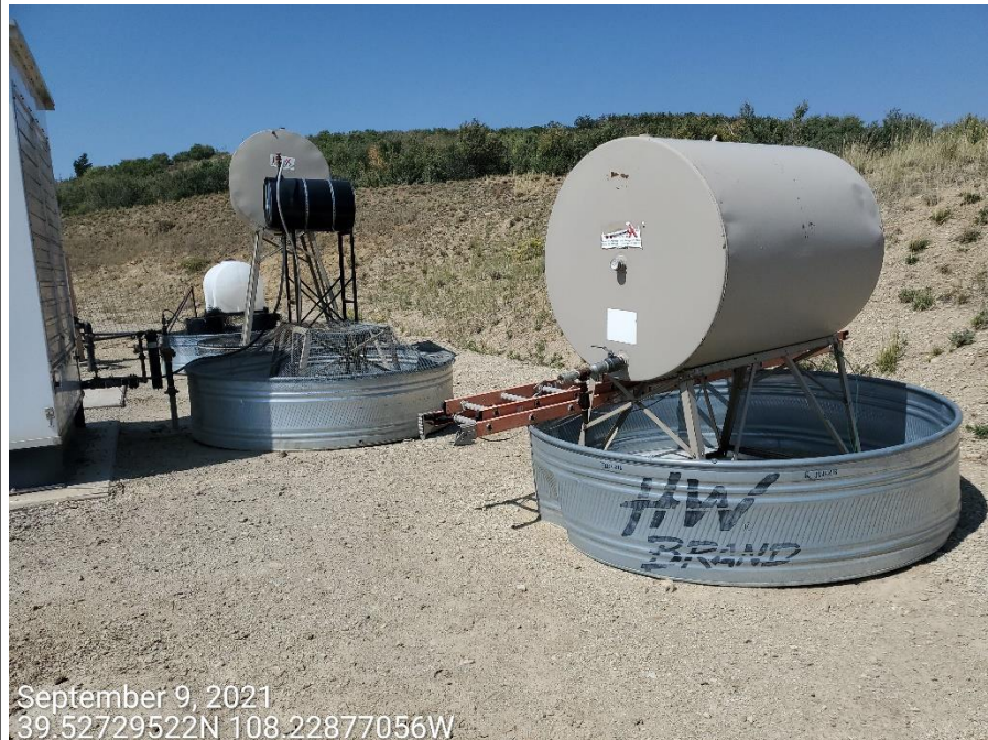
Photo 6: Photos provide examples showing that wildlife protection devices are missing or insufficient at several secondary containment BMPs.
