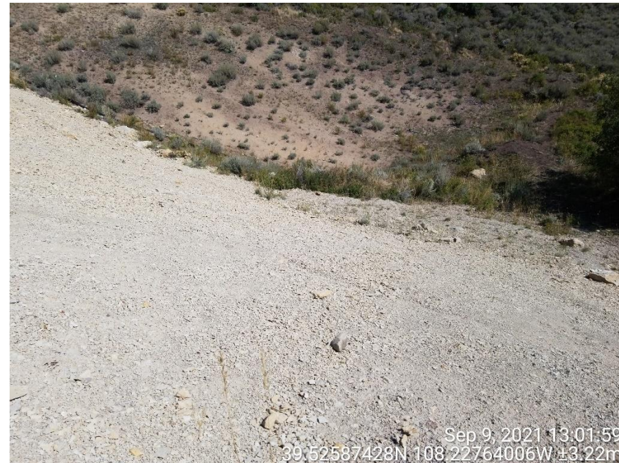
Photo 2: Photos taken from the fill slopes on the west end of the Location. Photos show BMPs to protect and stabilize the slopes, and manage runoff are missing or insufficient.
