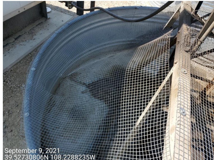
Photo 6: Photos provide examples showing that wildlife protection devices are missing or insufficient at several secondary containment BMPs.
