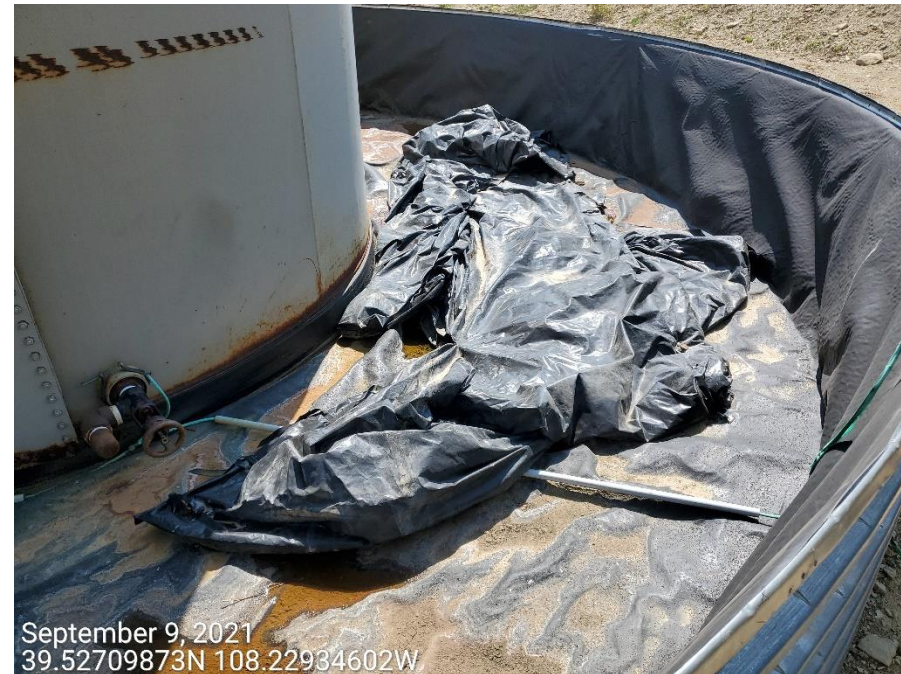
Photo 3: Photos provide example of various trash debris observed on areas north of the Location (photo left), and improperly stored within the secondary containment.
