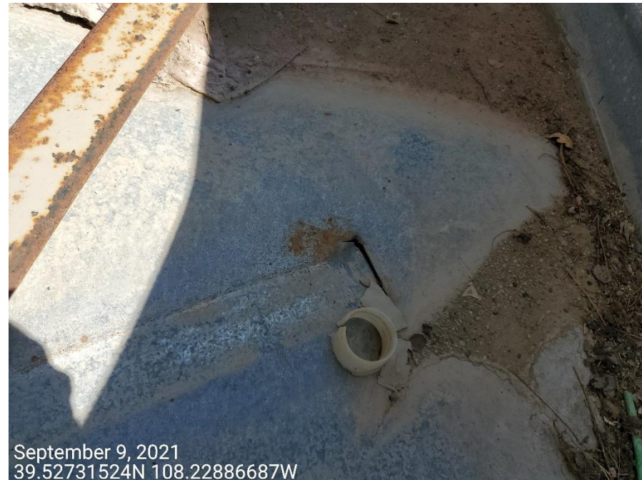
Photo 8: Photo taken from the containment BMP for the tank in left-photo 6. Photo shows multiple punctures observed at the base of the BMP.
