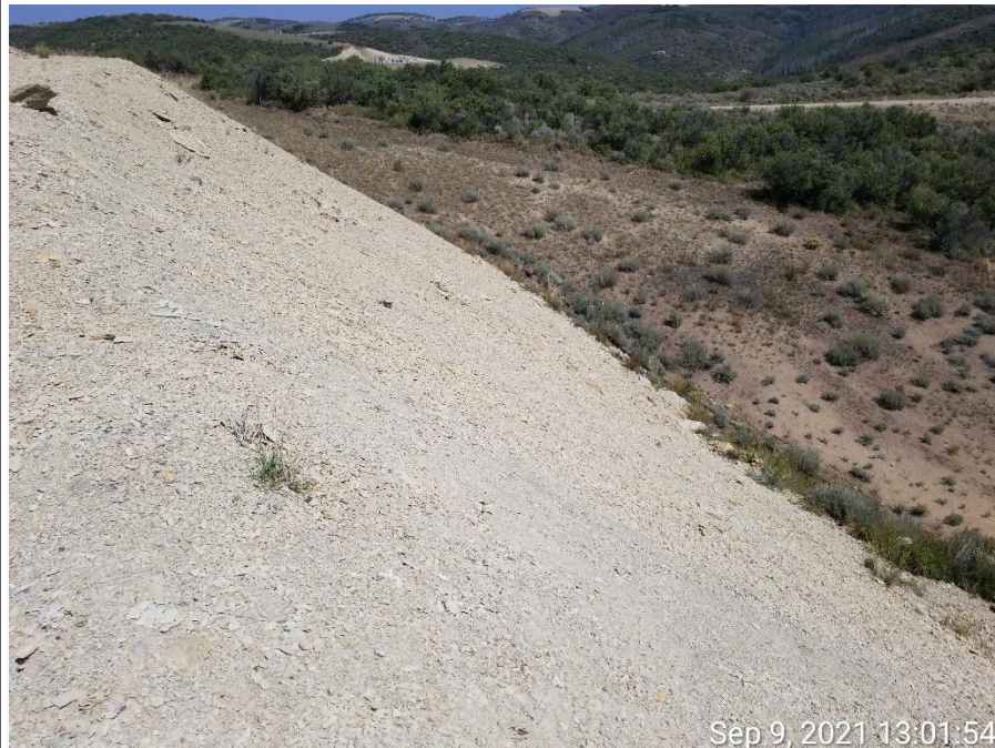
Photo 2: Photos taken from the fill slopes on the west end of the Location. Photos show BMPs to protect and stabilize the slopes, and manage runoff are missing or insufficient.
