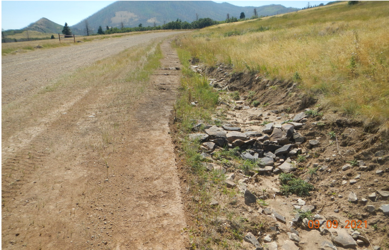
Photo 2. Facing southeast ascending the hill toward the location. There are rock check dams installed along the roadside.
