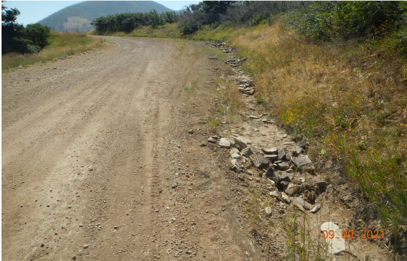
Photo 1. Facing southeast ascending the hill toward the location. There are rock check dams installed along the roadside. Some of the check dams will need maintenance.
