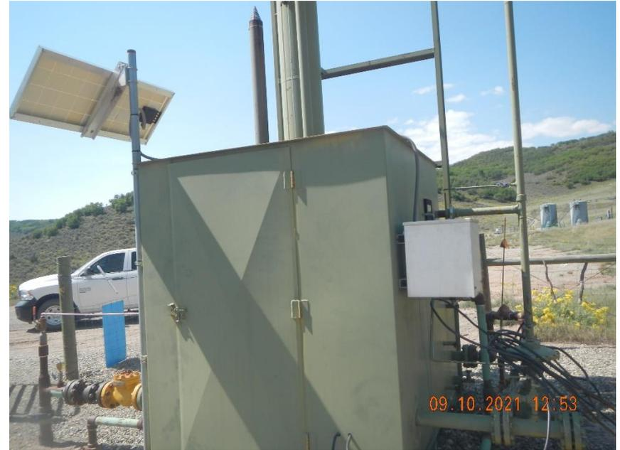
**Separator storage vessel contains no labeling**
