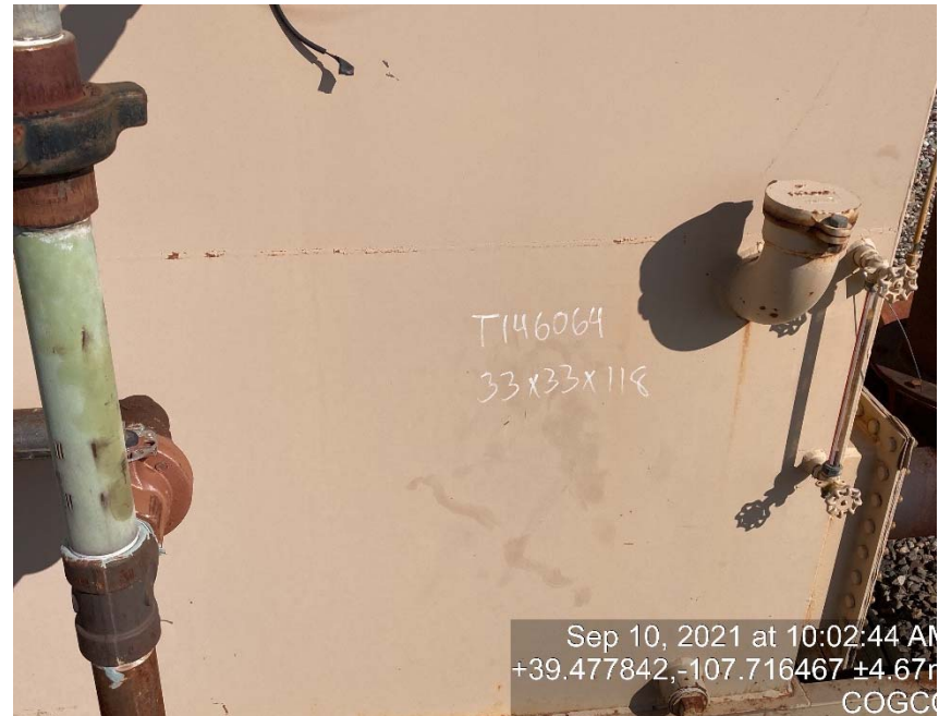
Dimensions of horizontal separator glycol storage vessel.
