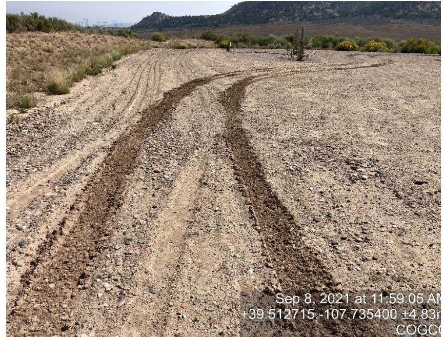
Lack of stabilization/compaction
