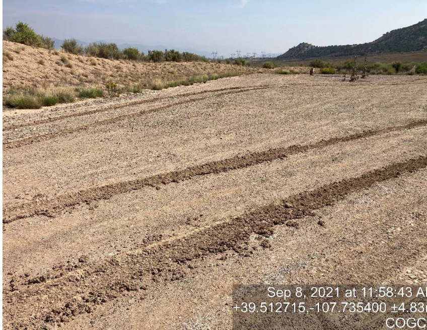
Lack of stabilization/compaction
