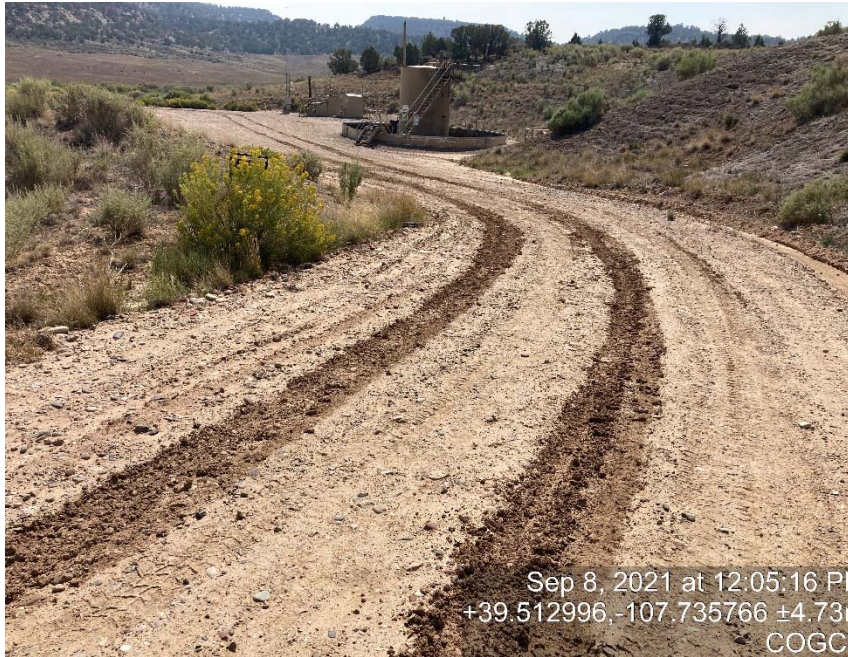
Lack of stabilization/compaction
