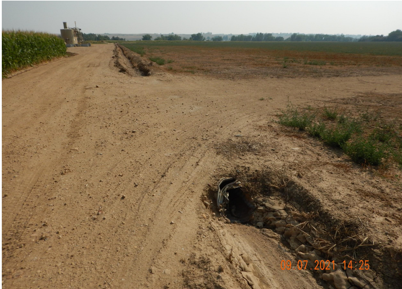
Photo 2. Photo taken from the entrance of the well location access road, facing South. Photo illustrates the culvert has not been removed.
