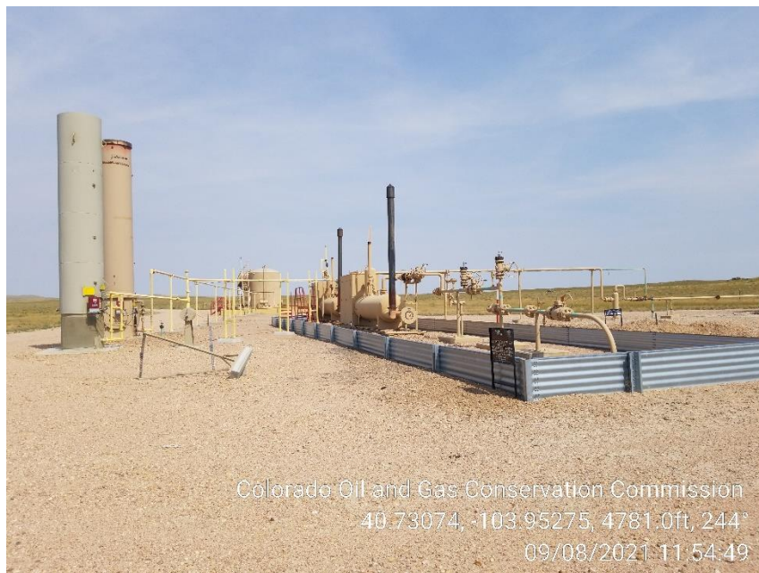
Photo 3 – Separators and ECDs
