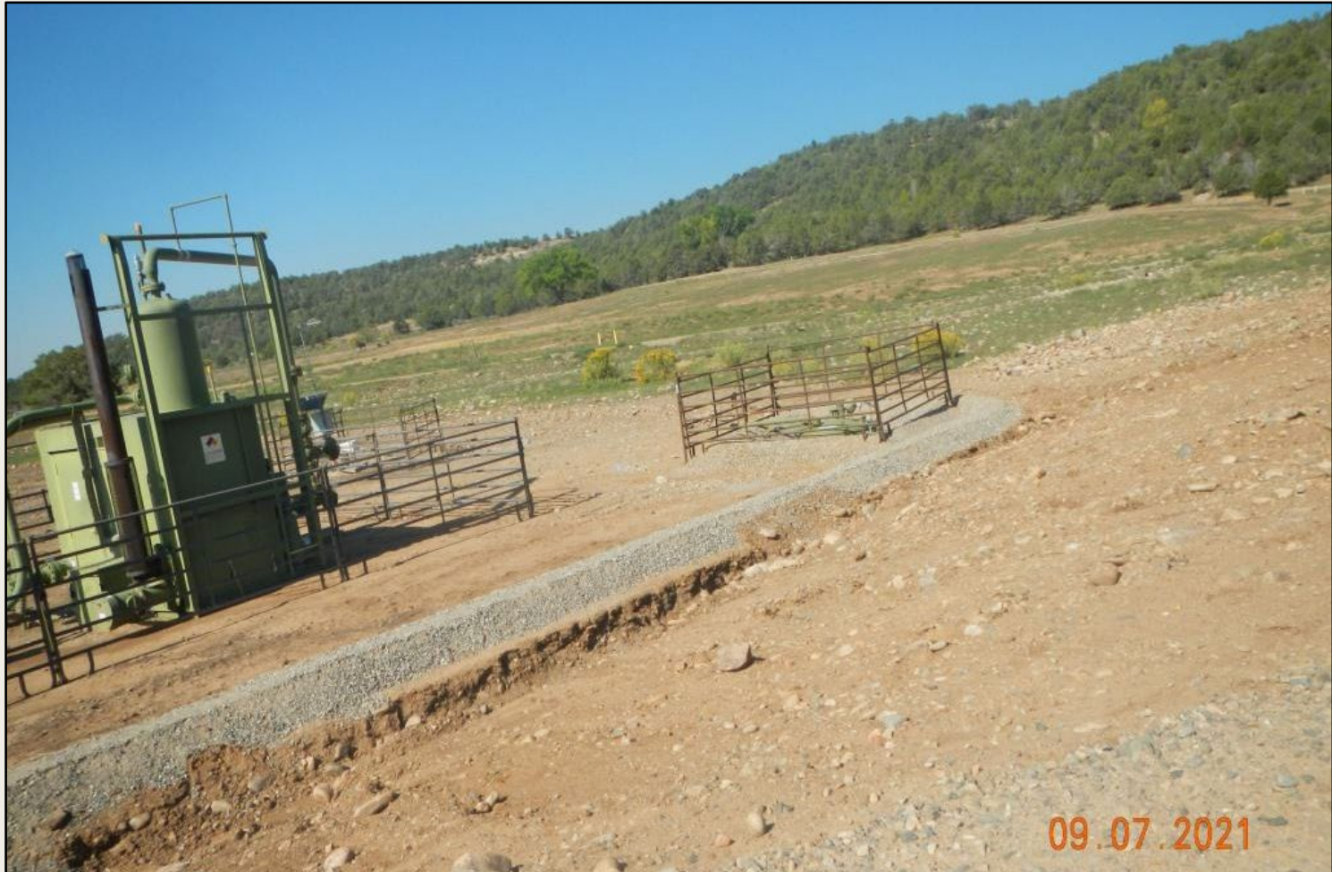
Photo 3. View of the northern project area facing westward. Well pad grading and berm construction is in process. Disturbed soils outside of the working area need seeding after work is completed.
