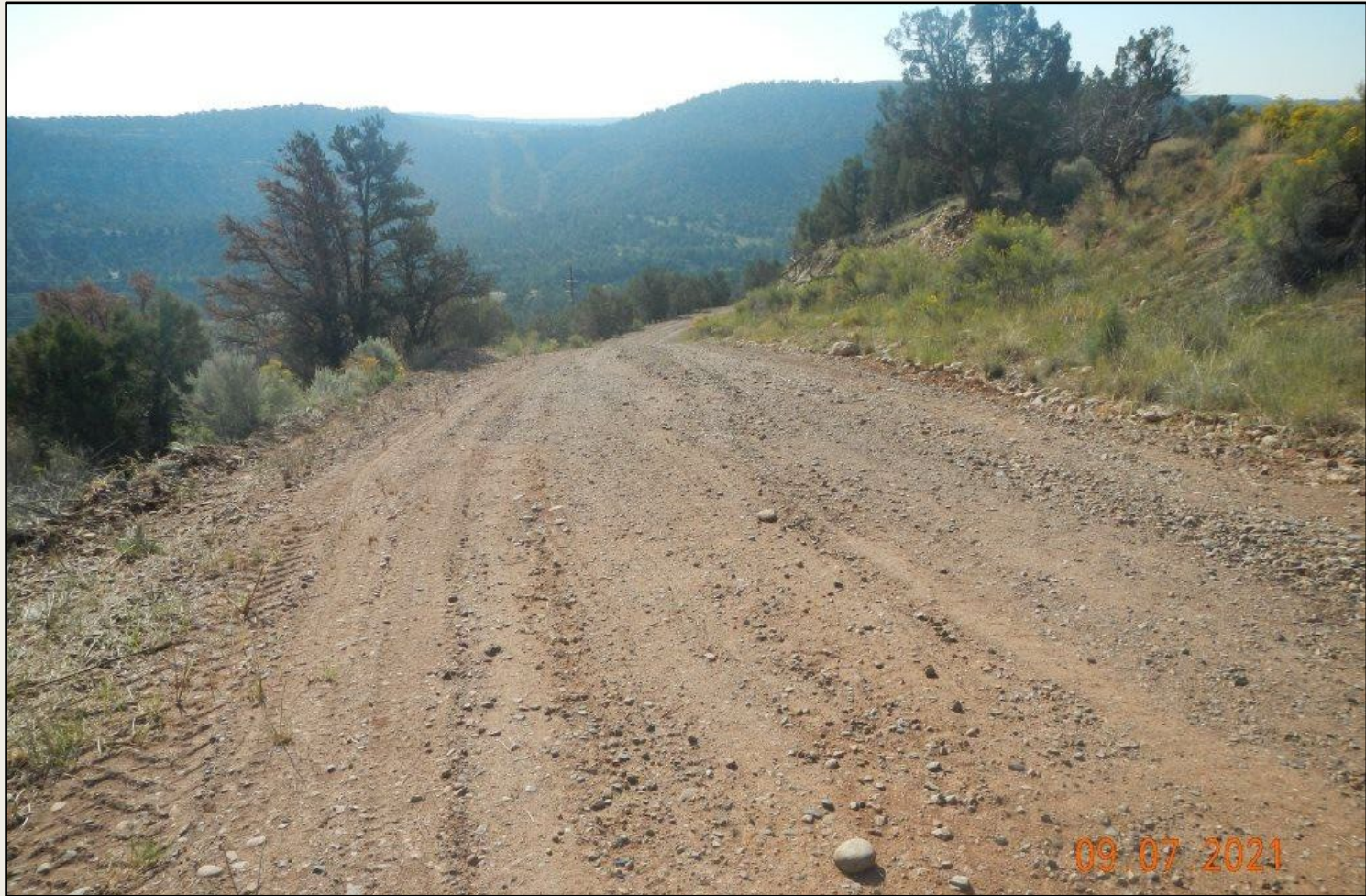
Photo 2. View of the access road, surface is recently graded, culverts and ditches are maintained.
