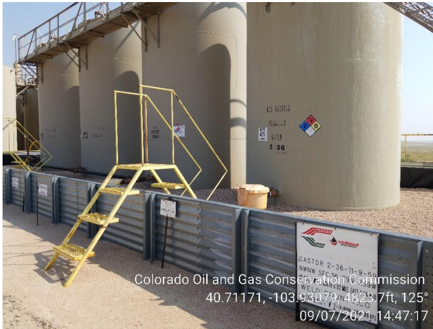
Photo 3 – Tank Battery
