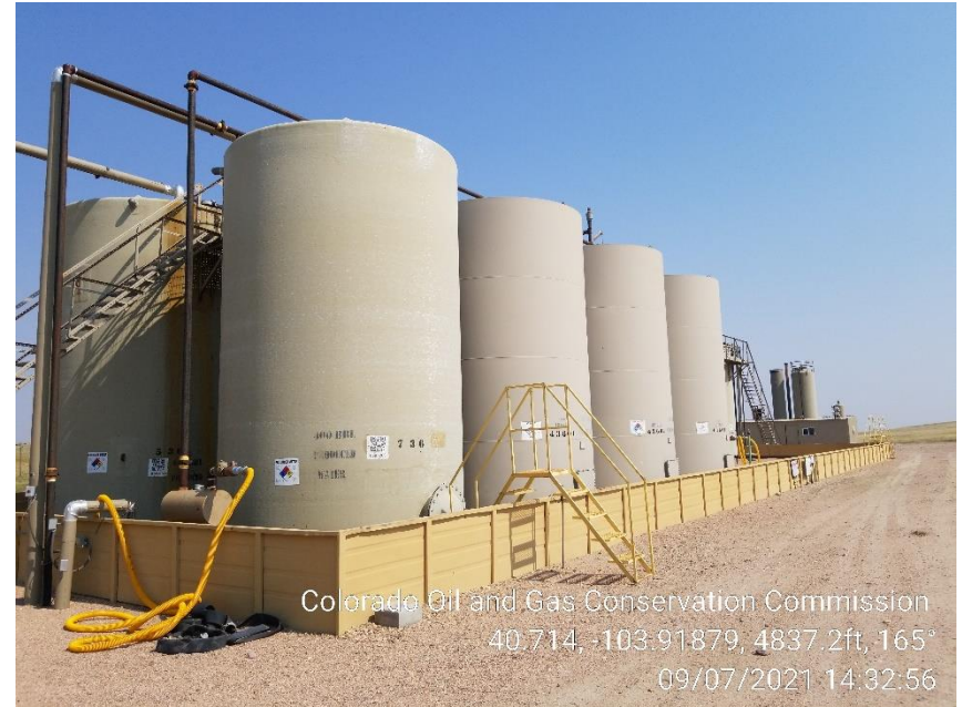
Photo 2 – Tank Battery
