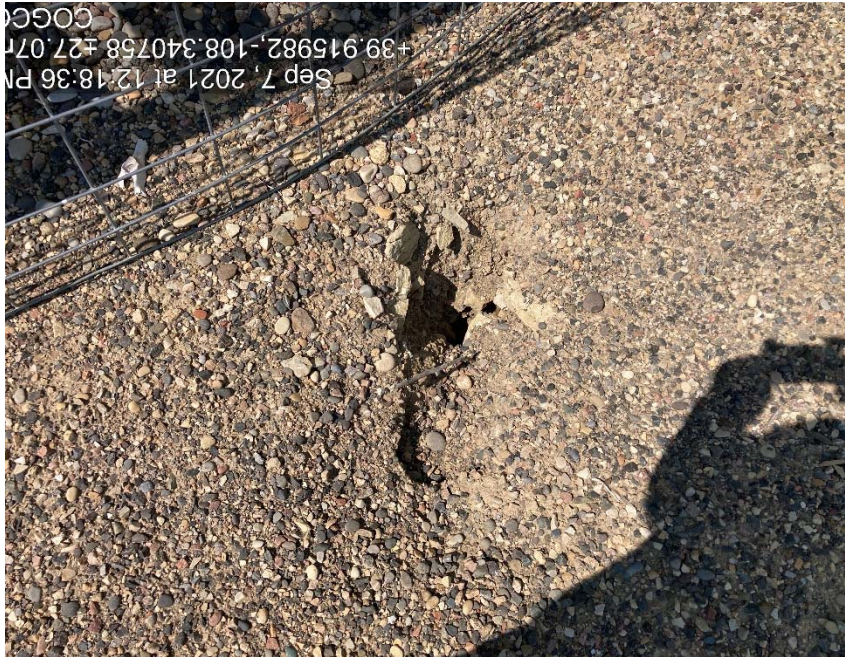
Subsidence at tank risers
