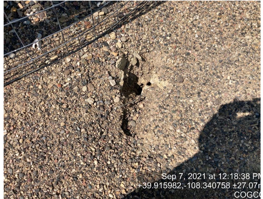
Subsidence at tank risers
