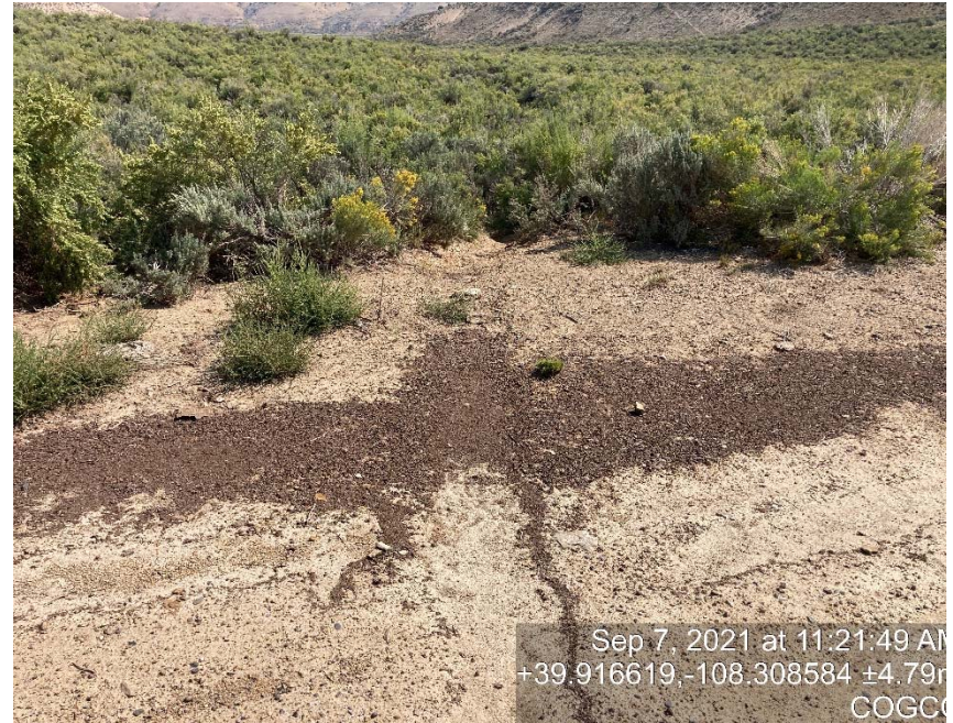
Sediment migration from pad next to separator
