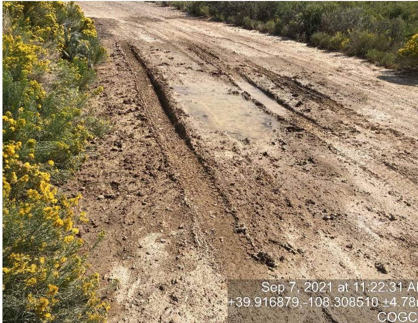
Lack of stabilization/compaction
