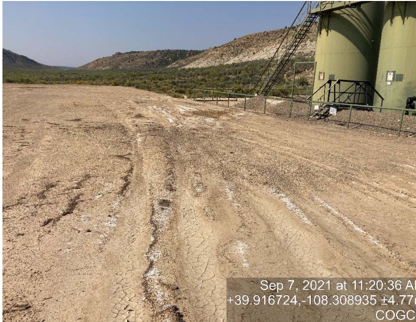
Lack of stabilization/compaction
