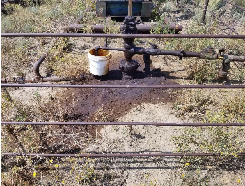
Photo 3. Stained soil at wellhead. No bradenhead access apparent.
